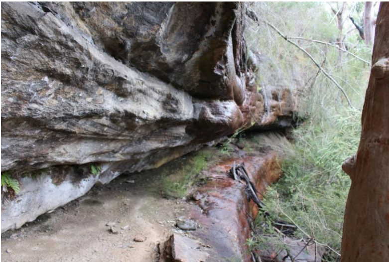
Plate 116: External context of FRC 195. View north.
