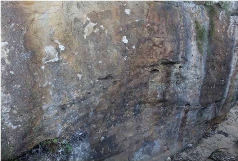
Plate 38: Overview of FRC 85, Panel 2. View east west.
