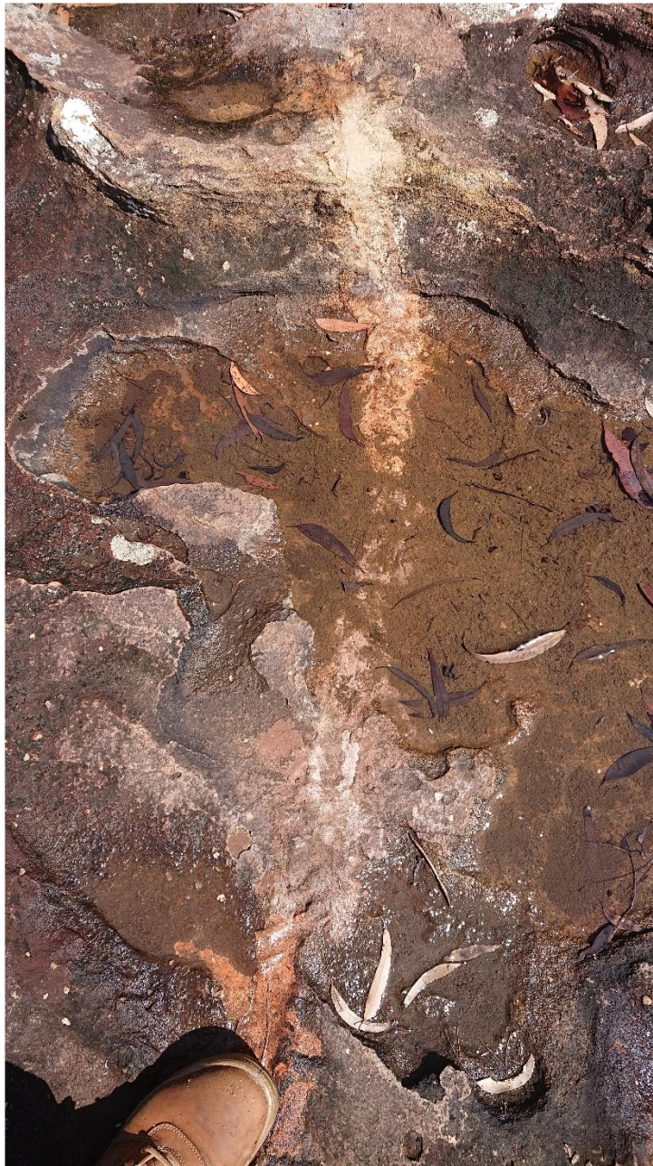
Photo 9 - Grout Curtain (Waratah Rivulet)
