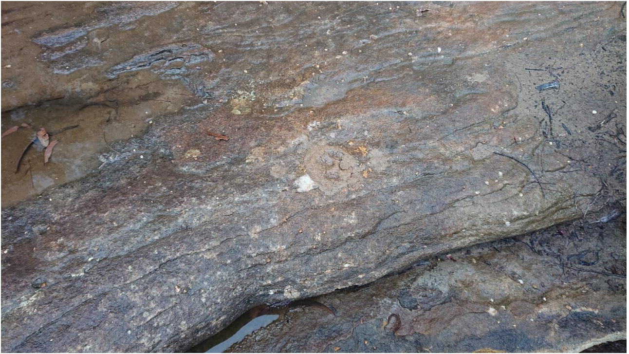
Photo 7 - Grout Injection Point (ETA H)
