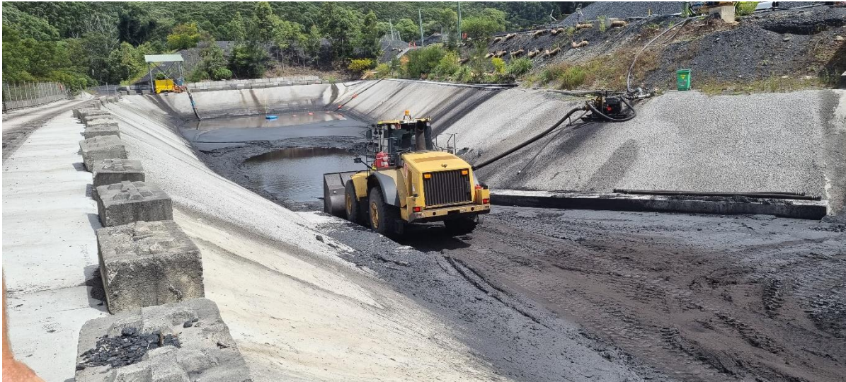
Photo 3 – Desilting the Turkeys Nest Sediment Pond
