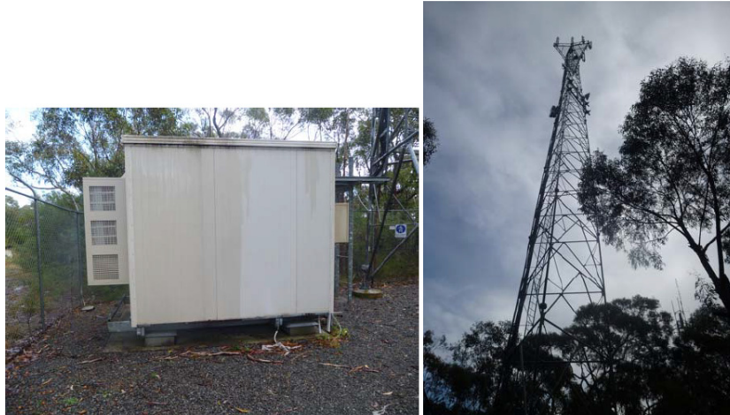
Plates 3 & 4 – Telecommunications Tower 2 and Compound (Source: MSEC, 2016)
