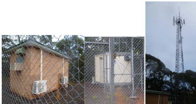
Plates 1 & 2 – Telecommunications Tower 1 and Compound (Source: MSEC, 2016)
