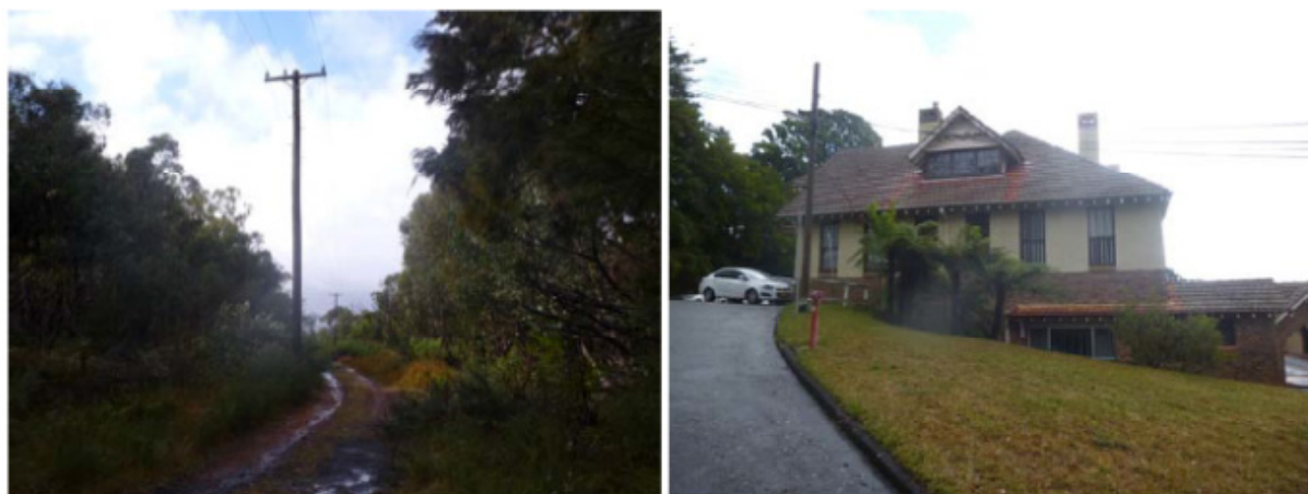
Plates 2 and 3 – Aerial Powerlines (Source: MSEC, 2016)
