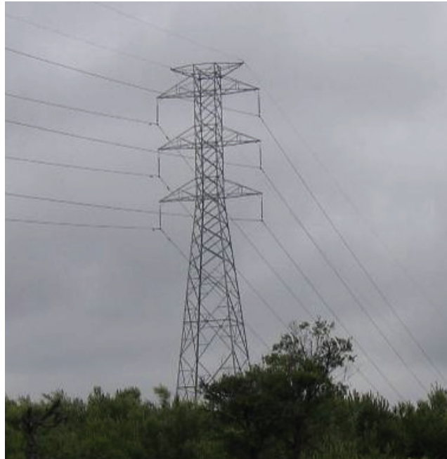
Figure 1 Photograph of a 132 kV Transmission Tower
