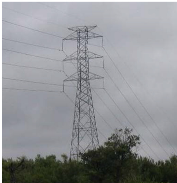
Plate 1 – 132 kV Transmission Tower (Source: MSEC, 2016)
