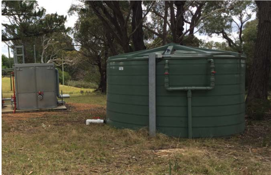
Figure 9 Water Storage Tanks Refs. B17t01 (poly tank) and B18t01 (steel tank)
