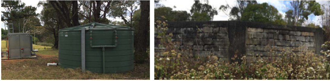
Plates 17 & 18 – Fire Water Tank and Steel Tank Adjacent Pump House, and Trickle Filter Tank (Source: MSEC, 2016)
