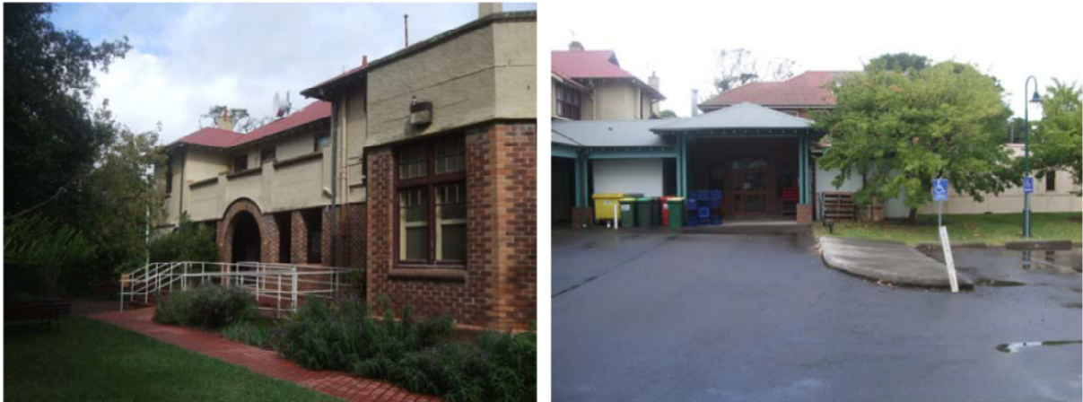
Plates 7 & 8 – Aged Care Building Structures [B01e] {Nurses Quarters} (Source: MSEC, 2016)
