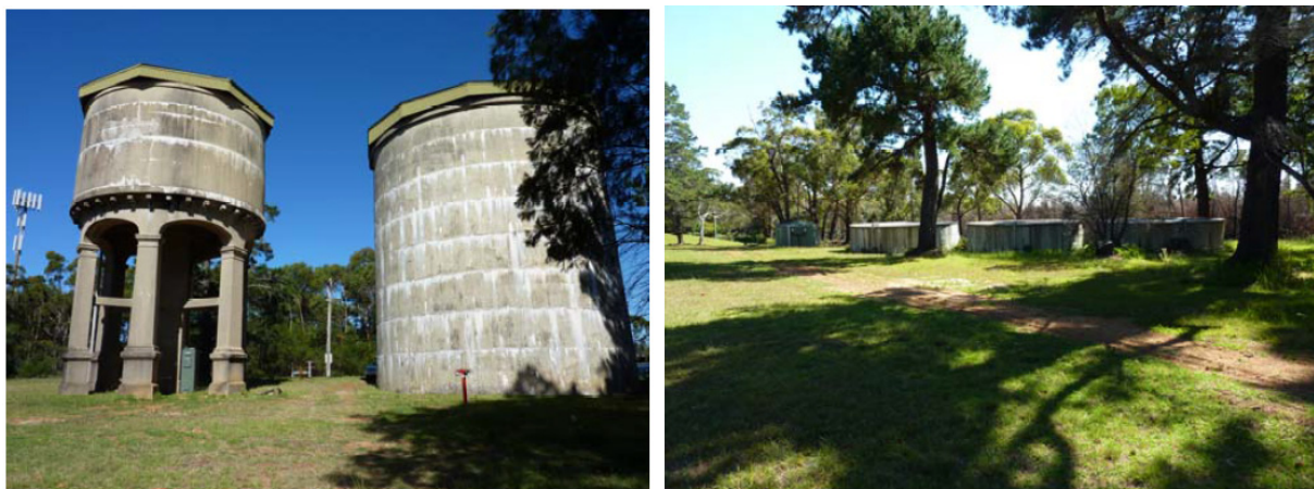
Plates 15 & 16 – Large Water Storage Tanks (Source: MSEC, 2016)
