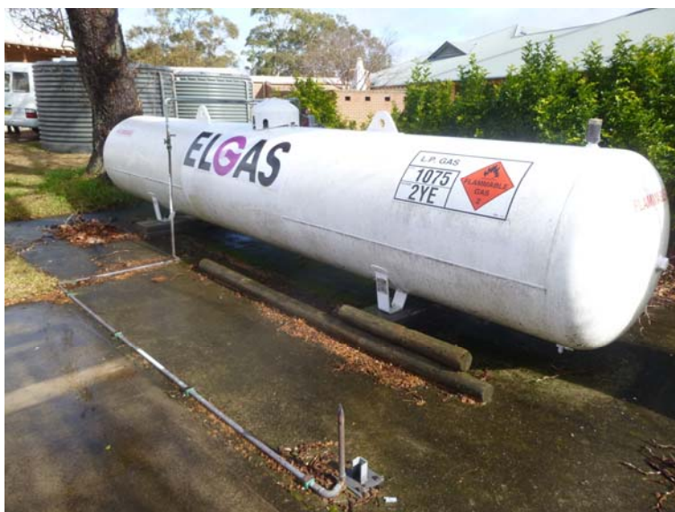
Figure 10 Gas Storage Tanks Refs. B01t03 and B01t04
