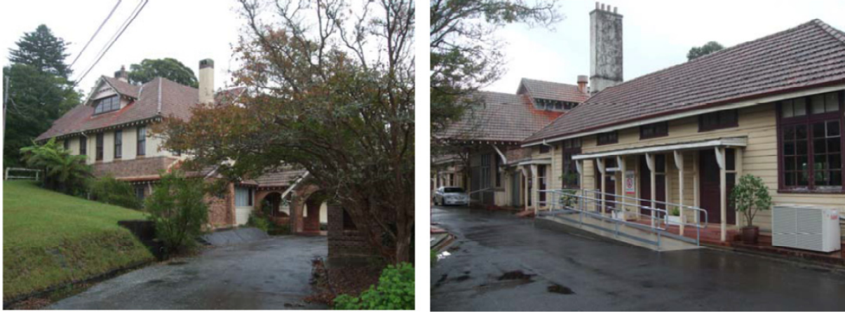
Plates 9 & 10 – Aged Care Building Structures [B02a & B02b] {Administration/Kitchen Group} (Source: MSEC, 2016)
