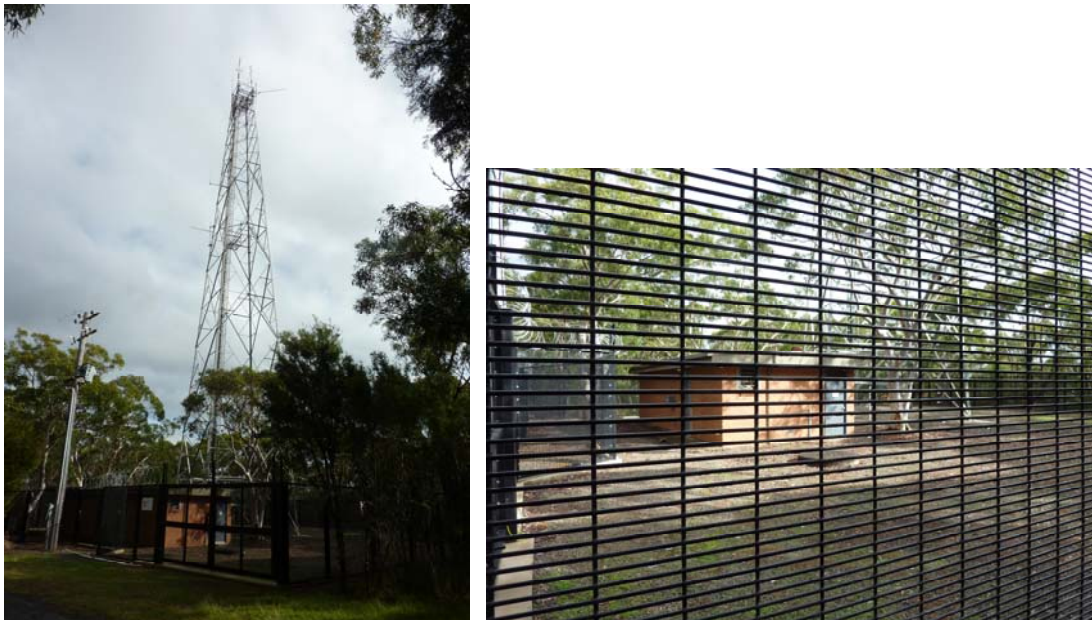
Figure 1 Telecommunications Tower and Compound
