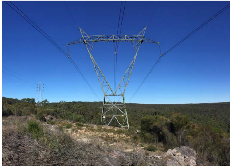
Plate 1 – 330 kV Transmission Tower (Source: MSEC, 2016)
