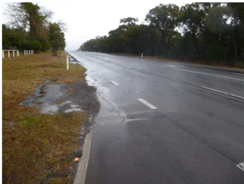
Plate 1 – Old Princes Highway (Source: MSEC, 2016)
