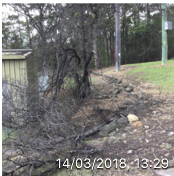
Vent Shaft Stormwater
