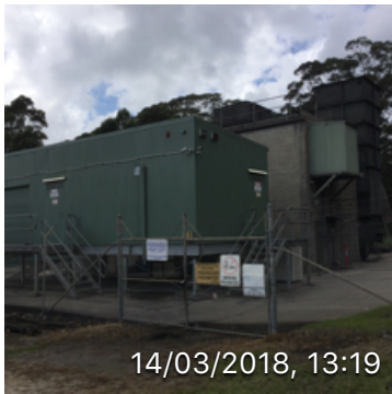
Mine Vent Shaft
