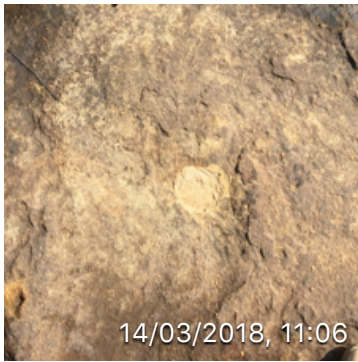
Poly Urethane injection point
