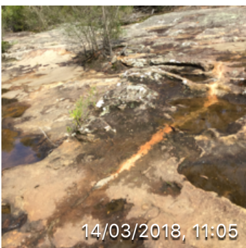
Poly Urethane Grout filled crack near Pool F
