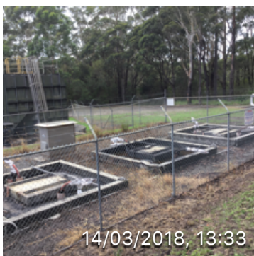
Vent Shaft Transformer Pads
