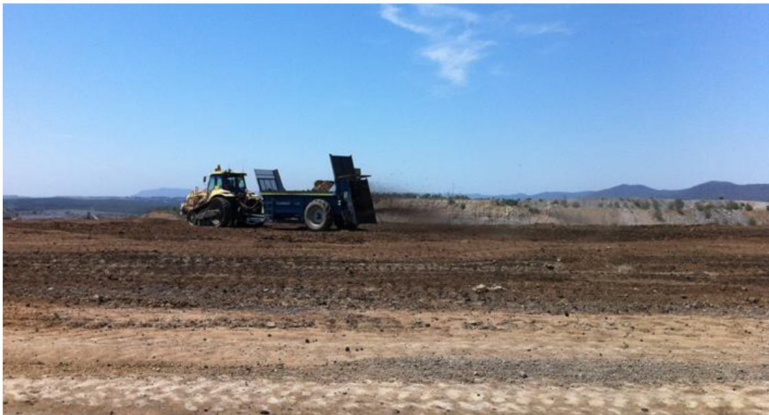
Plate 1 – Biosolid Application on Re-profiled Waste Rock Emplacement
