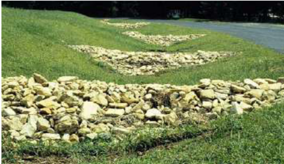
Figure 7: Example of Check Dams
