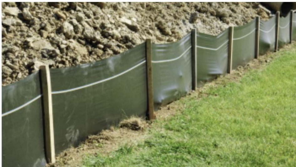
Figure 6: Example of Sediment Fencing
