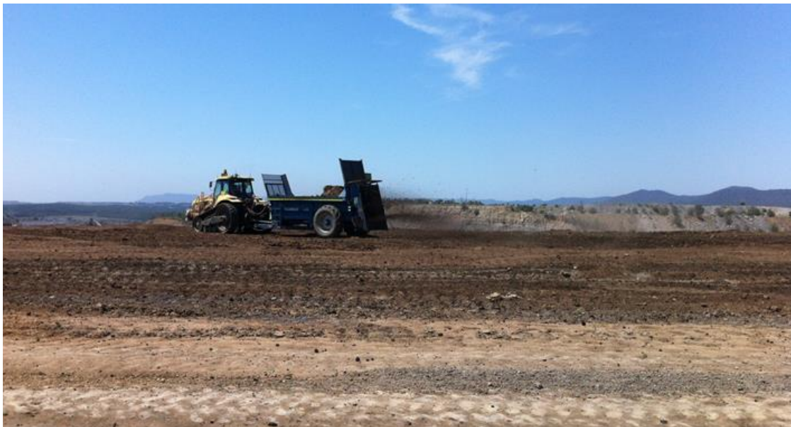
Plate 1 – Biosolid Application on Re-profiled Waste Rock Emplacement
