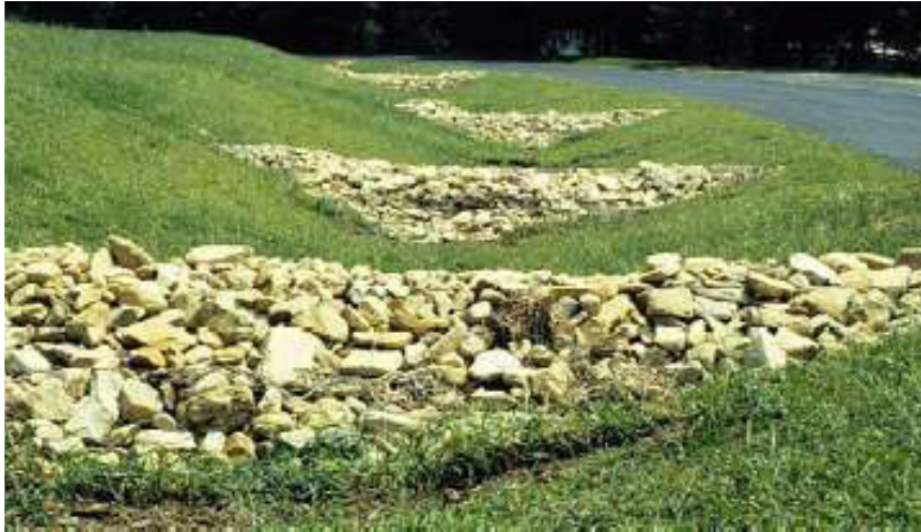
Figure 7: Example of Check Dams
