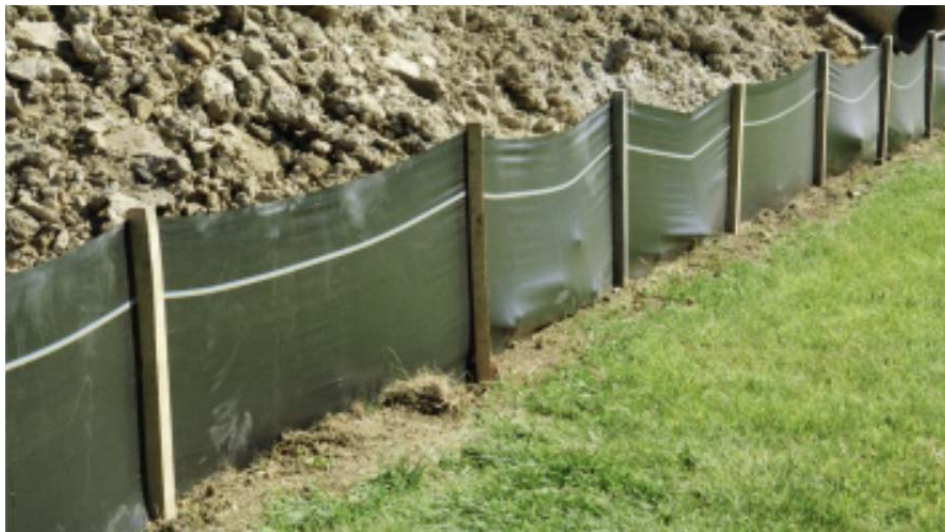
Figure 6: Example of Sediment Fencing
