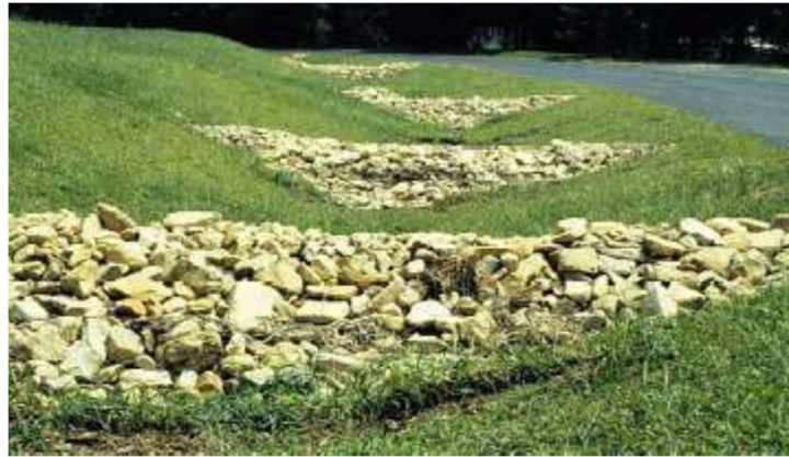
Figure 8: Example of Check Dams
