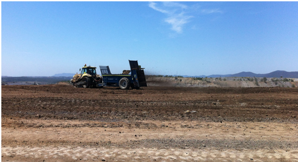
Plate 1 – Biosolid Application on Re-profiled Waste Rock Emplacement
