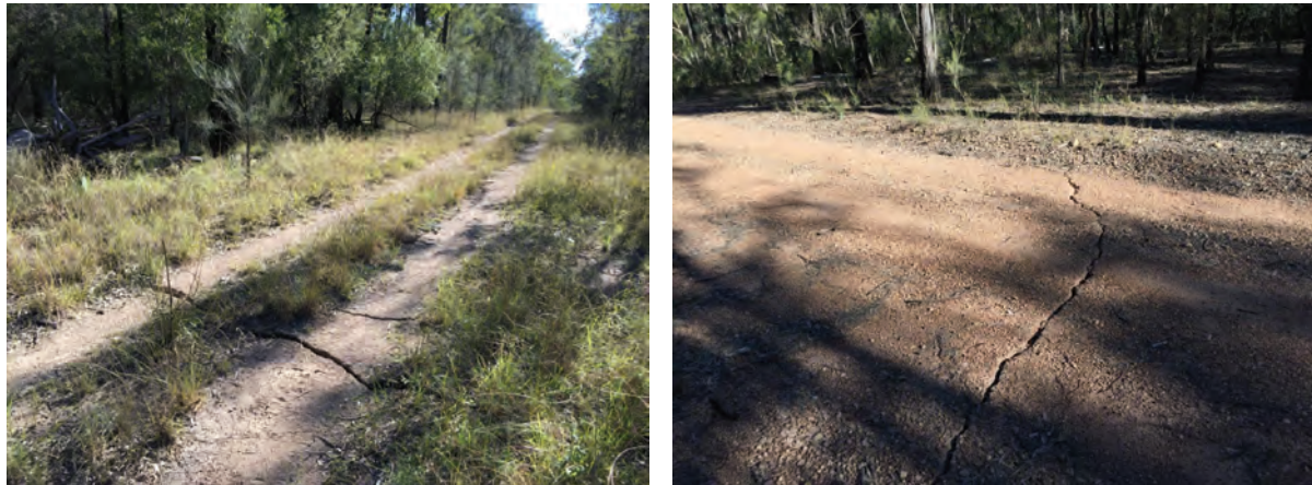
Fig. 4.9 Cracking along the access tracks above the central part of WYLLW13 (Source: WCPL)
