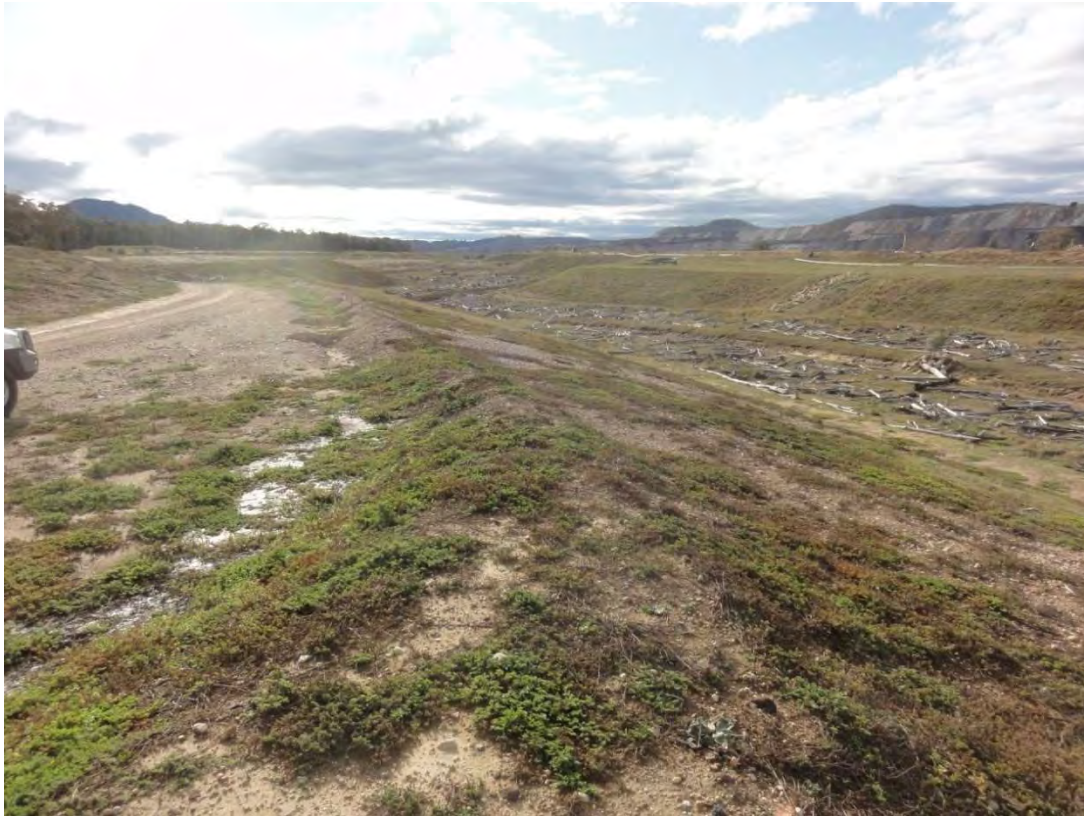
Figure 2-13. Typical conditions in mid Stage 3 of NWCD
