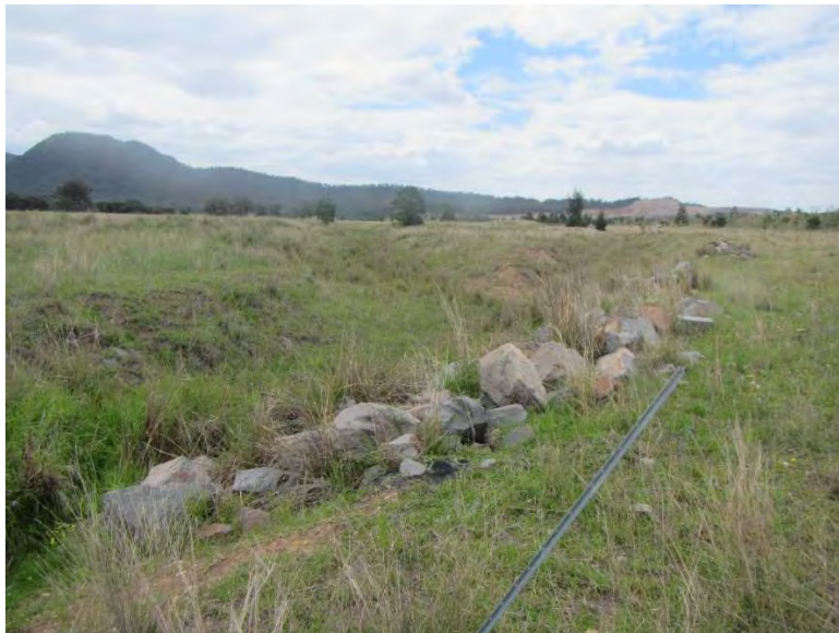
Figure D-0- 3. Rock beaching along existing outlet to NWCD (outlet 1)
