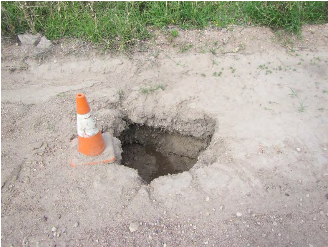
Figure 3-2 - Tunnelling over LW12/15 on track adjacent diversion
