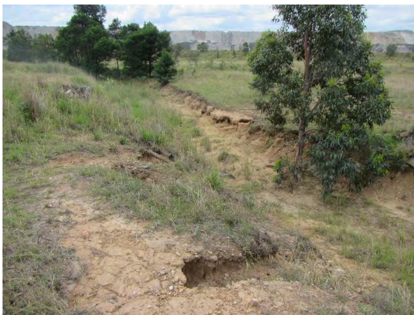
Figure D-0- 6. NWCD at base of proposed batter chute location
