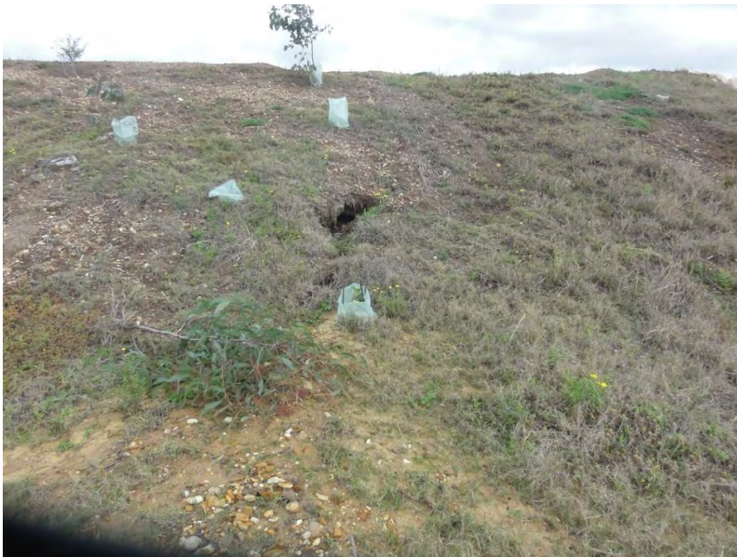
Figure 2-14. Tunnel erosion associated with overland flow management in Stage 3 NWCD is the subject of a management program by Wambo Coal
