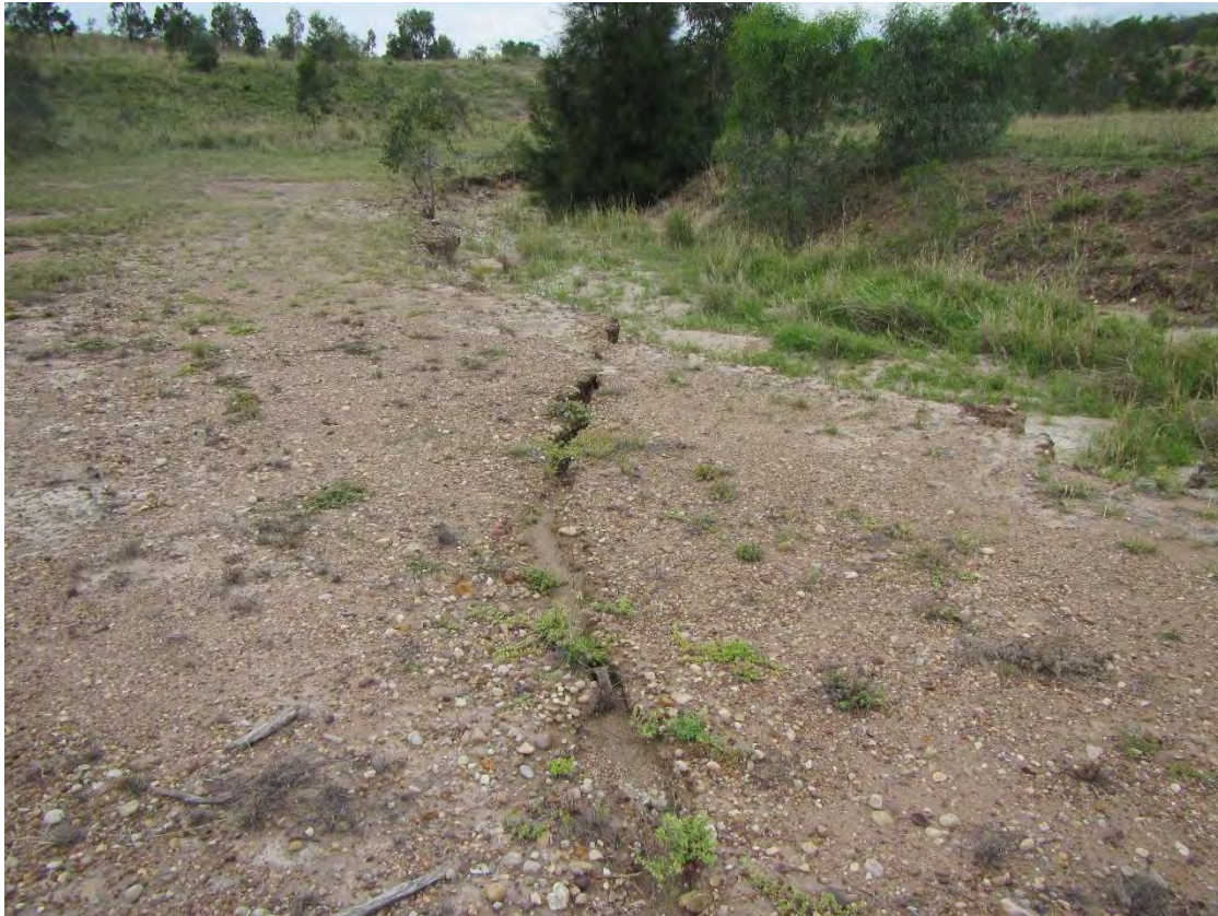
Figure 2-8. Cracking in inset floodplain over LW 11 in dispersive soils may lead to new tunnel and gully erosion
