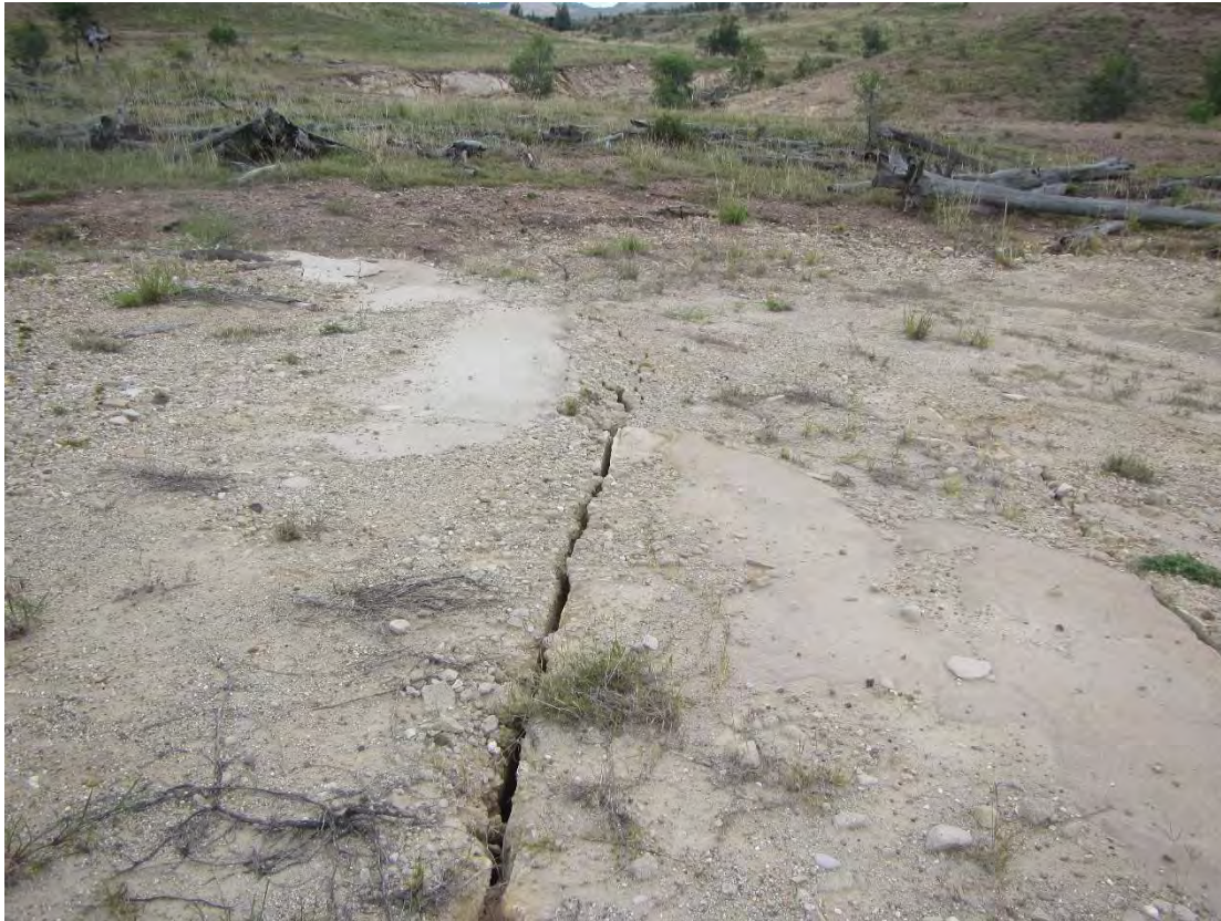
Figure 2-11. Compression buckle cracks at 1-2m spacing through the sandstone in NWCD near Div8 over LW 13/14
