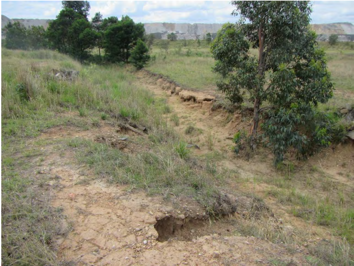
Figure 2-6. Minor overland flow and bank erosion in dispersive soils, mid stage 2 NWCD near Div3
