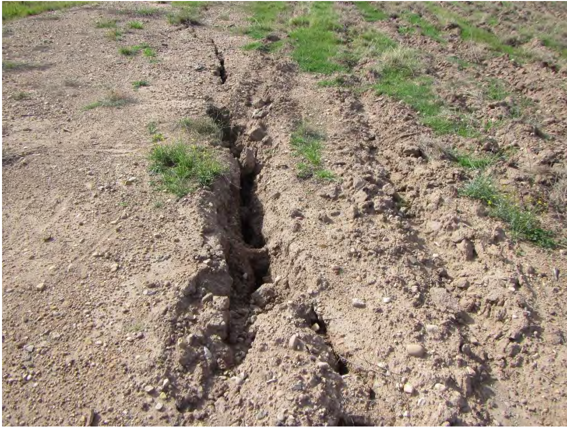
Figure 3-1 - Cracking at surface over LW13/14
