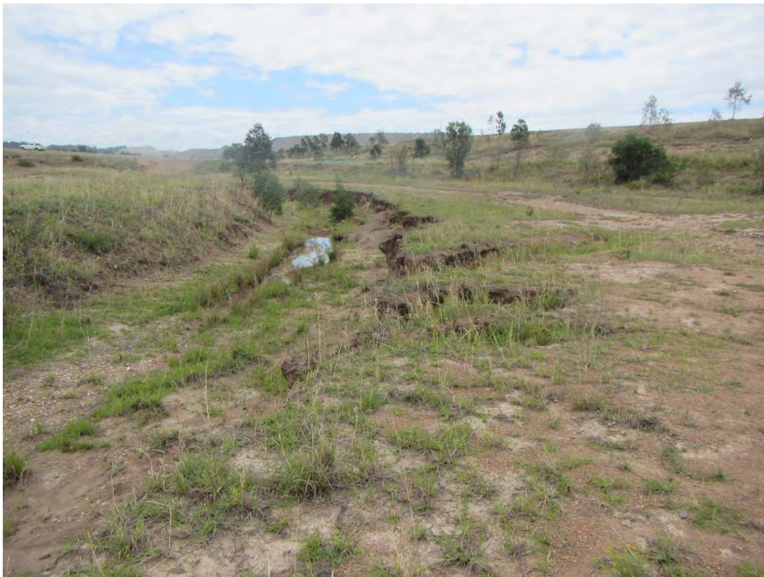
Figure 2-7. Section of NWCD Stage 2 near Div 5 already undergoing erosional adjustment that will be subject to increased erosion risk from LW 11-16 subsidence
