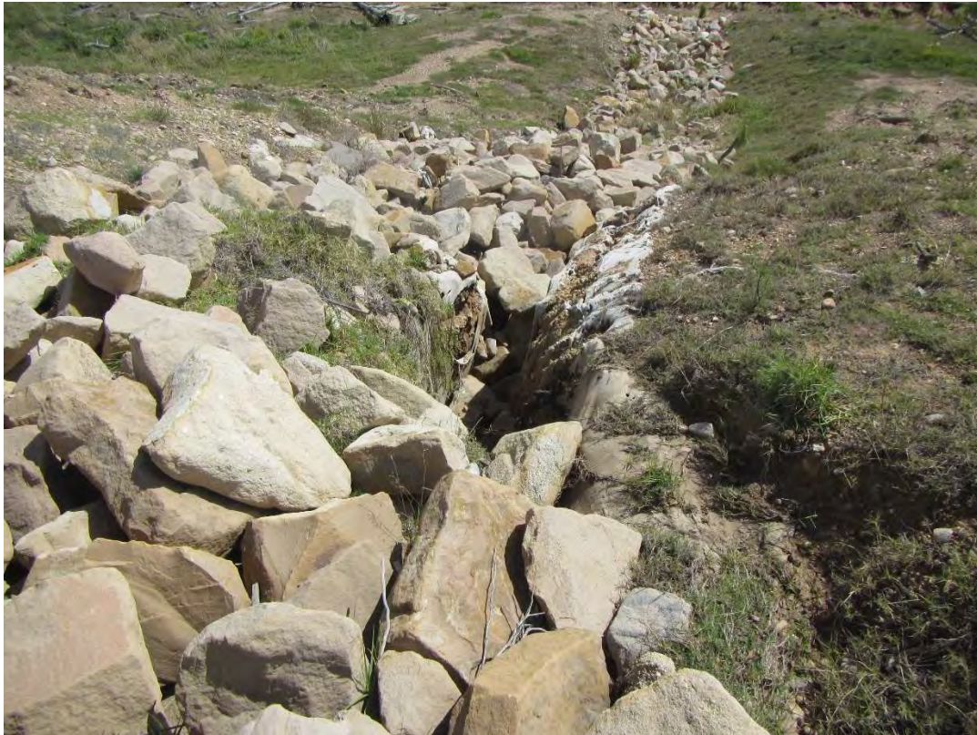
Figure 2-15. Tunnel erosion undermining one of the overland flow entry structures that requires management
