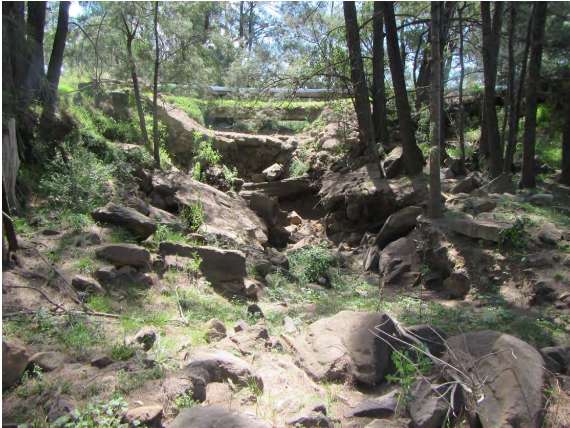
Figure 2-22. A significant step in bed profile through culverts near downstream extent of North Wambo Creek
