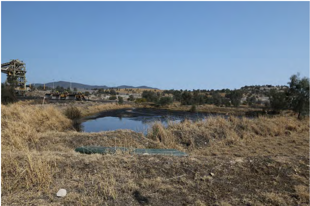
Plate 8 Coal Sediment Accumulation at the Gordon Below Franklin Storage
