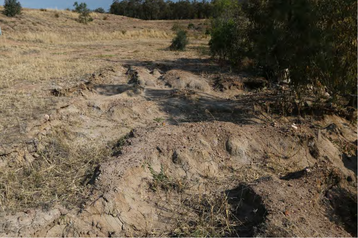
Plate 3 Example of Erosion on Stage 2 of the North Wambo Creek Diversion
