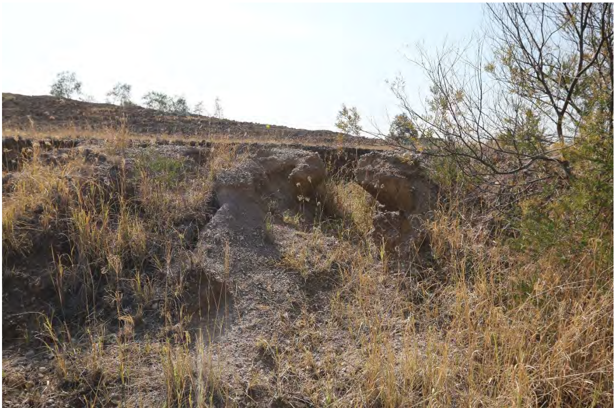
Plate 2 Example of Erosion on Stage 2 of the North Wambo Creek Diversion
