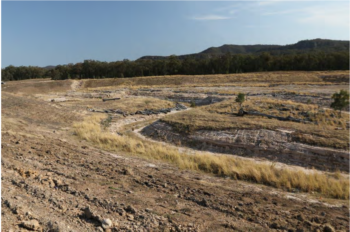
Plate 5 Bedrock Exposure on Stage 3 of the North Wambo Creek Diversion
