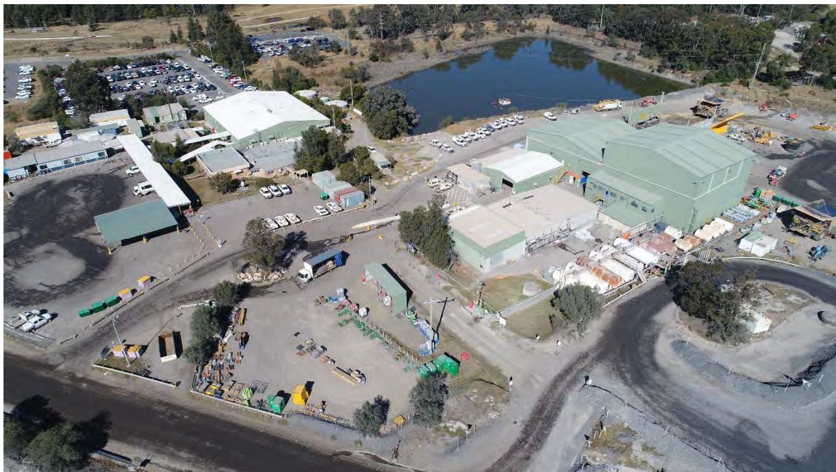
Plate 1 Administration and OC Workshop
