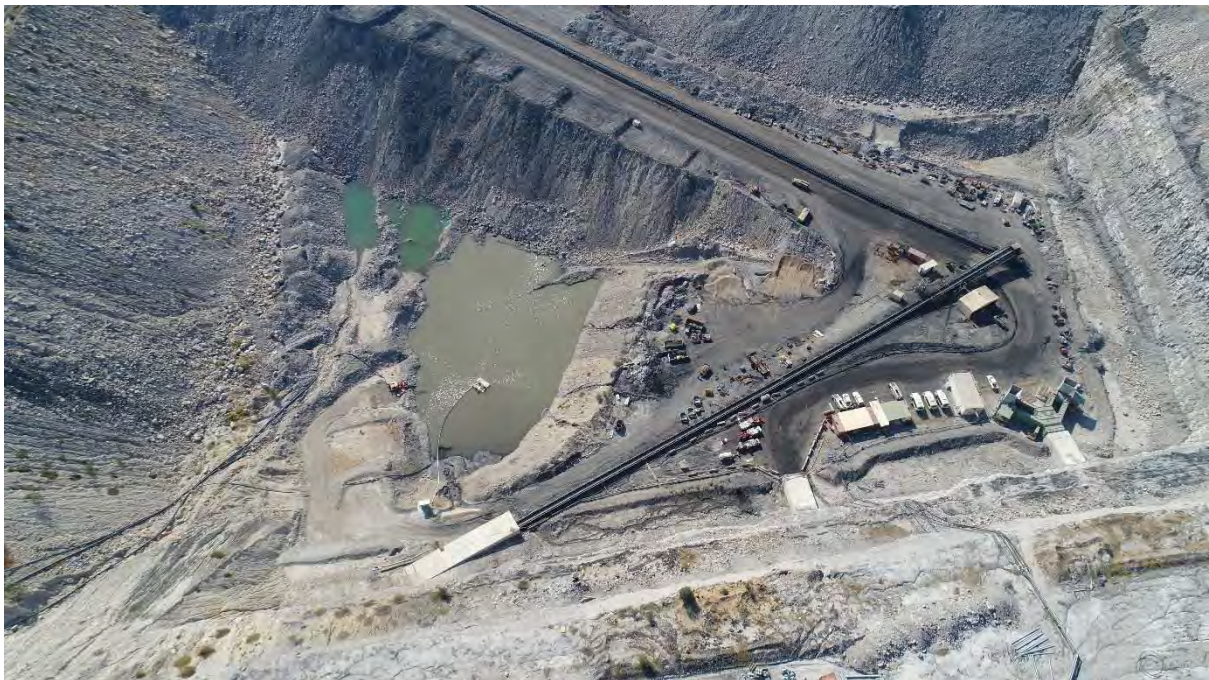
Plate 6 South Bates Underground
