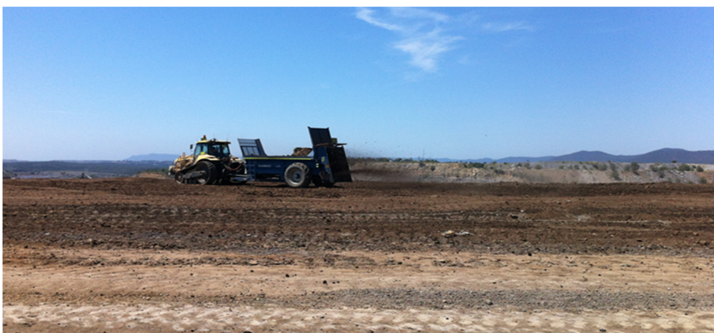
Plate 1 – Biosolid Application on Re-profiled Waste Rock Emplacement
