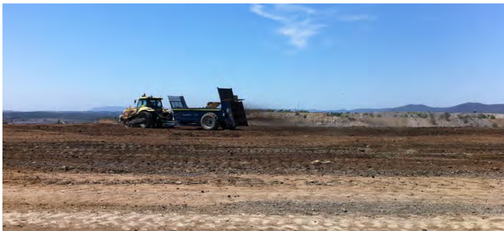
Plate 1 – Biosolid Application on Re-profiled Waste Rock Emplacement
