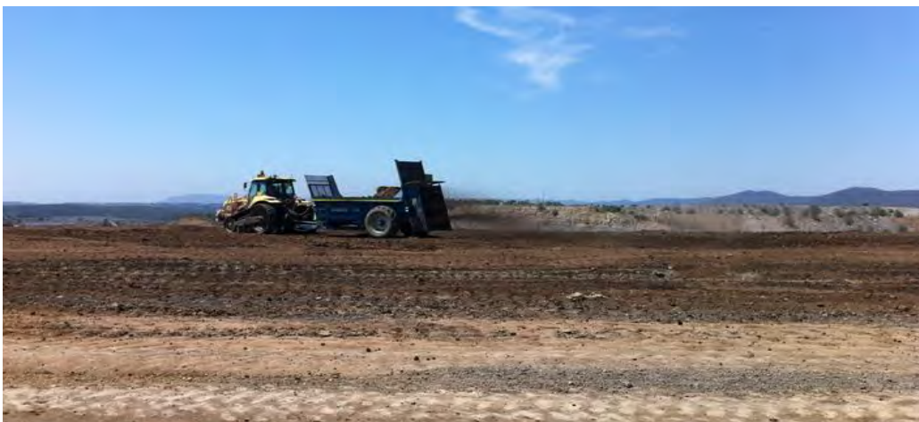
Plate 1 – Biosolid Application on Re-profiled Waste Rock Emplacement
