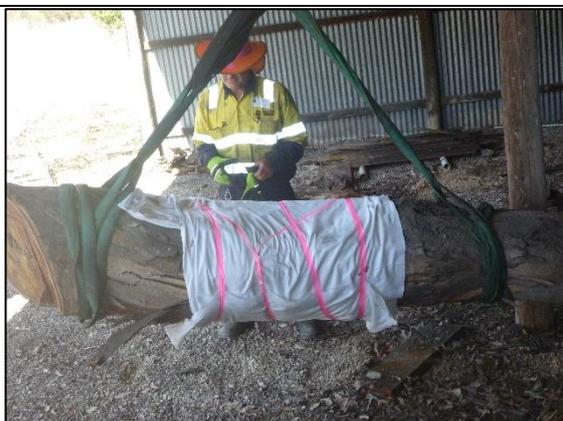
Figure 52 WCP113 wrap over scar and beginning lift
