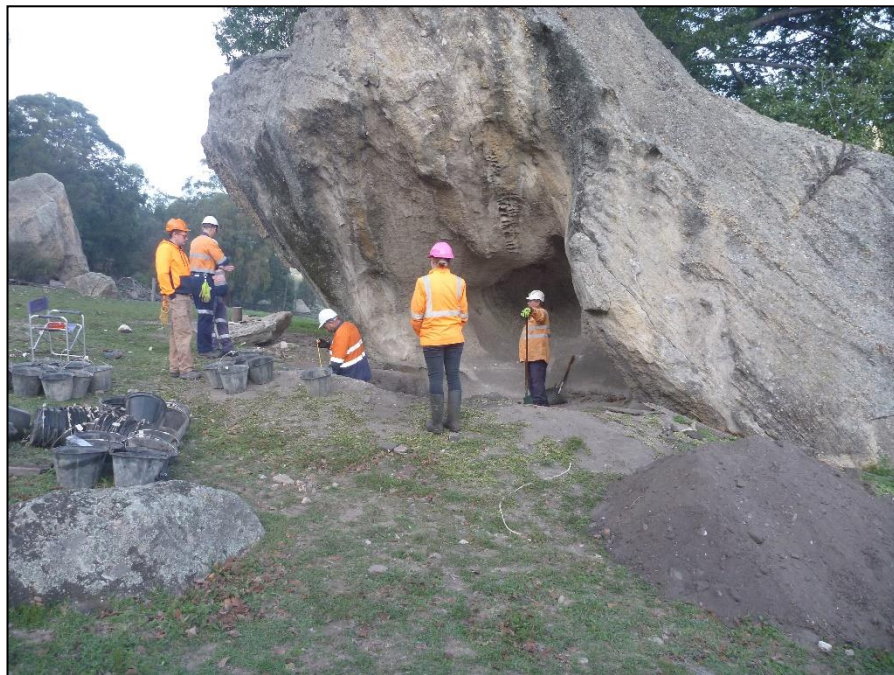
Figure A19 Cultural salvage works at WCP118. The stockpile of soil from the top ~50cm of 100 and 101 and the front of the mound is evident in the front left of the photo.
