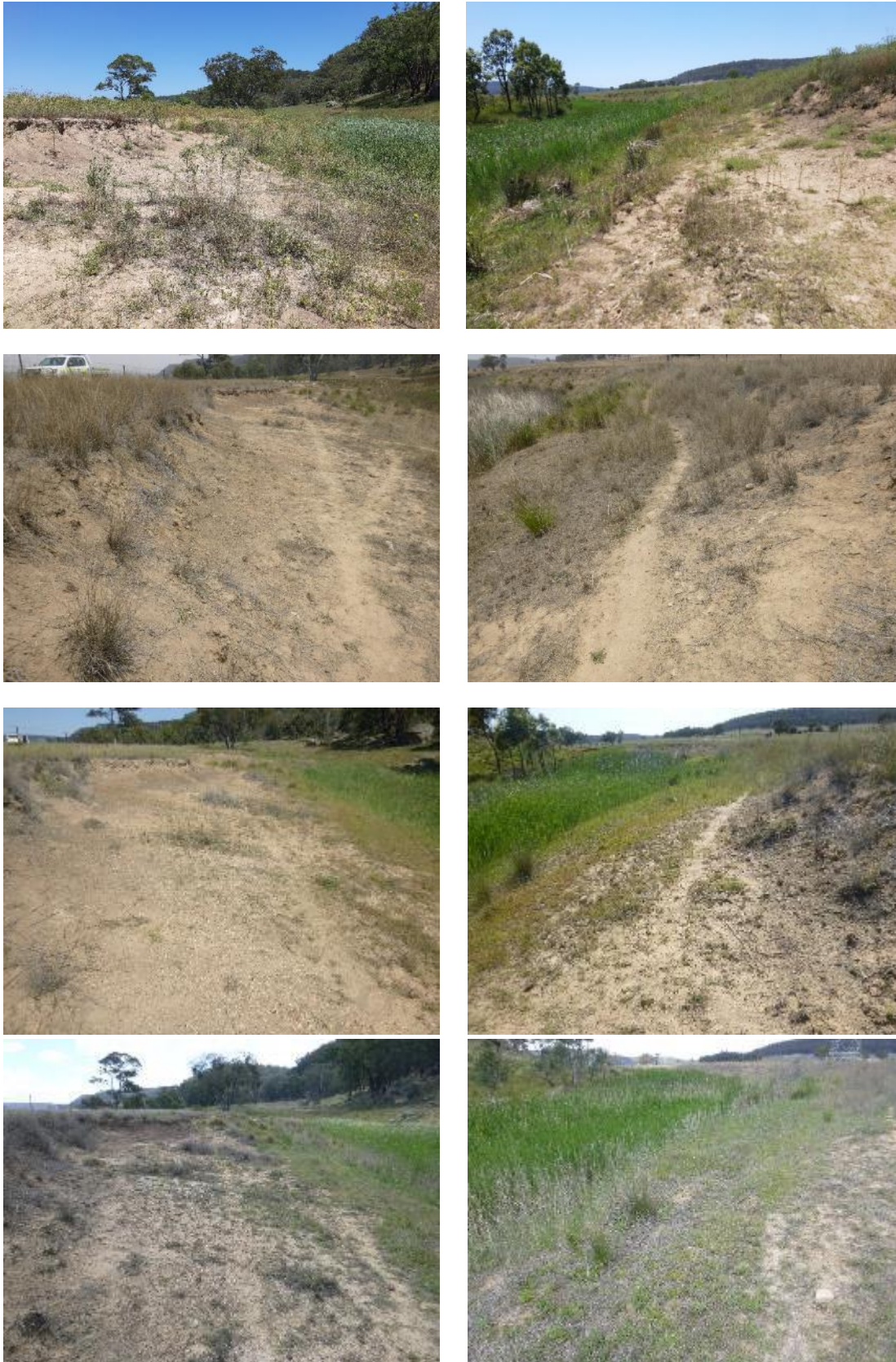
Figure B - 35: Wck35 site photos clockwise from top left: 2020 upstream, 2020 downstream, 2019 downstream, 2018 downstream, 2017 downstream, 2017 upstream, 2018 upstream, 2019 upstream
