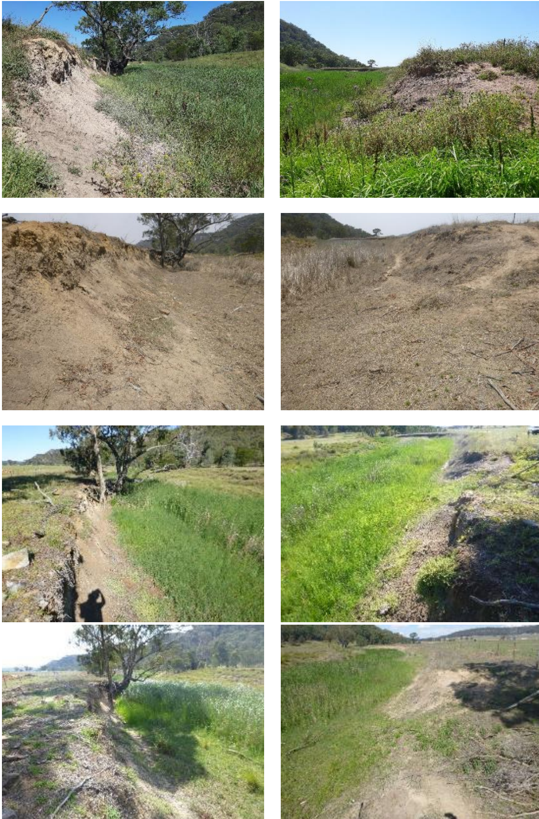
Figure B - 32: Wck32 site photos clockwise from top left: 2020 upstream, 2020 downstream, 2019 downstream, 2018 downstream, 2017 downstream, 2017 upstream, 2018 upstream, 2019 upstream
