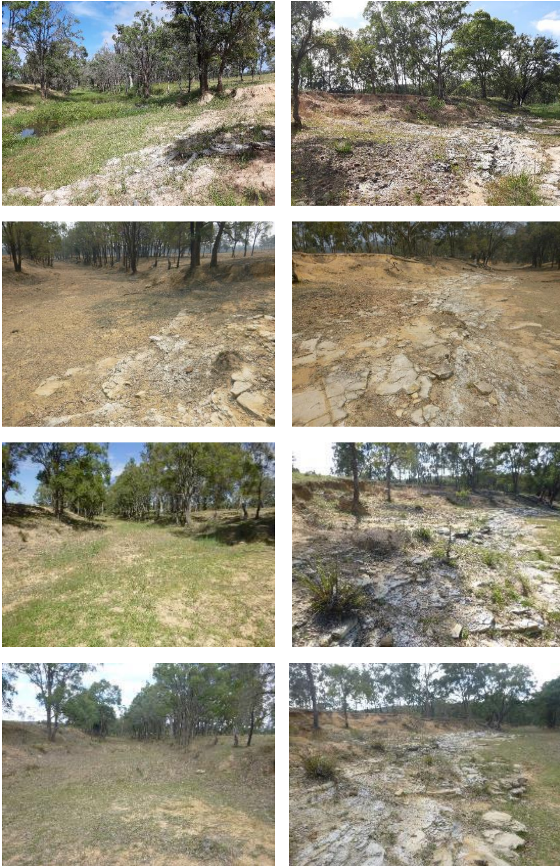
Figure B - 3: Wck3 site photos clockwise from top left: 2020 upstream, 2020 downstream, 2019 downstream, 2018 downstream, 2017 downstream, 2017 upstream, 2018 upstream, 2019 upstream
