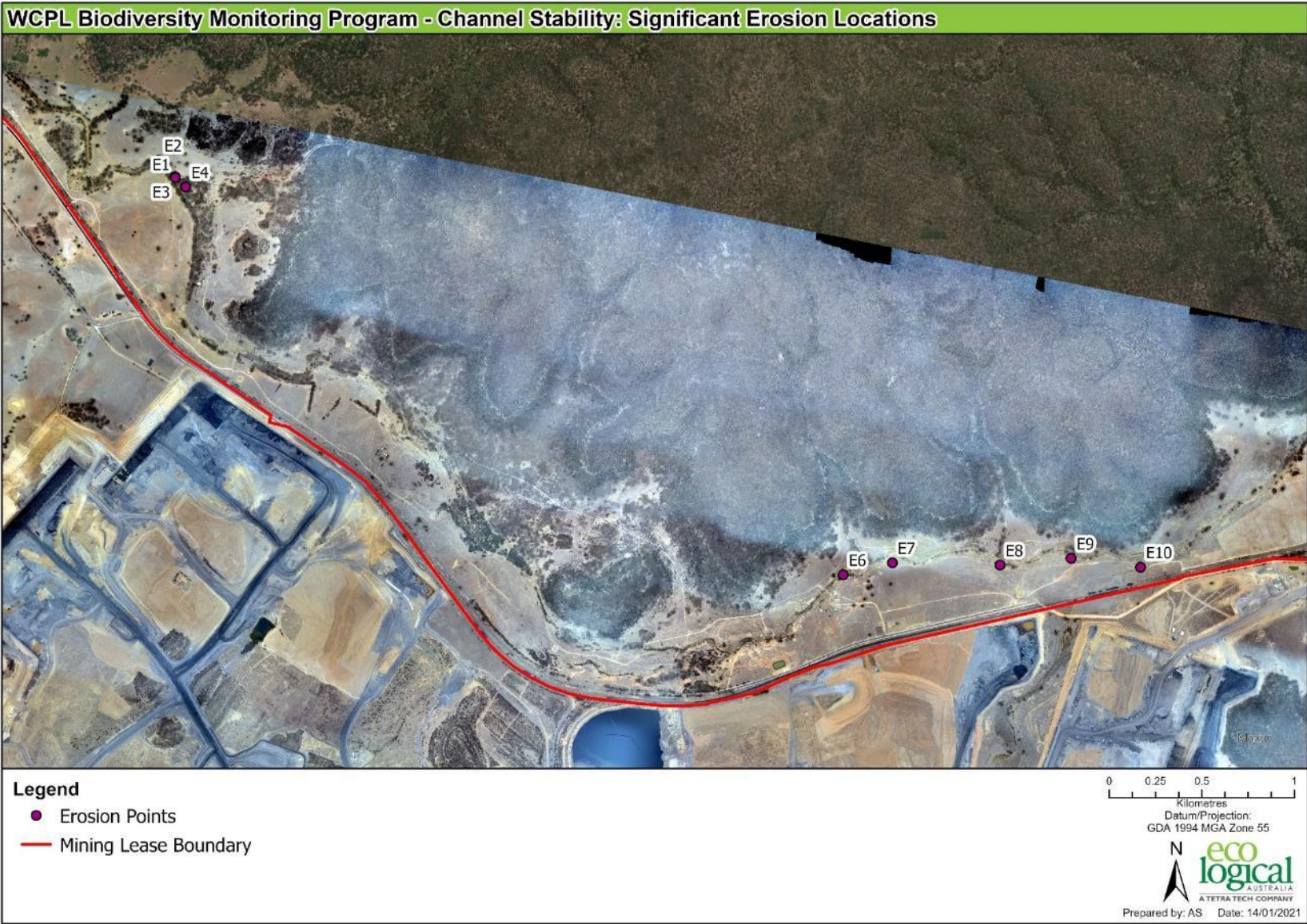
Figure 2: Significant erosion locations along Wilpinjong Creek
