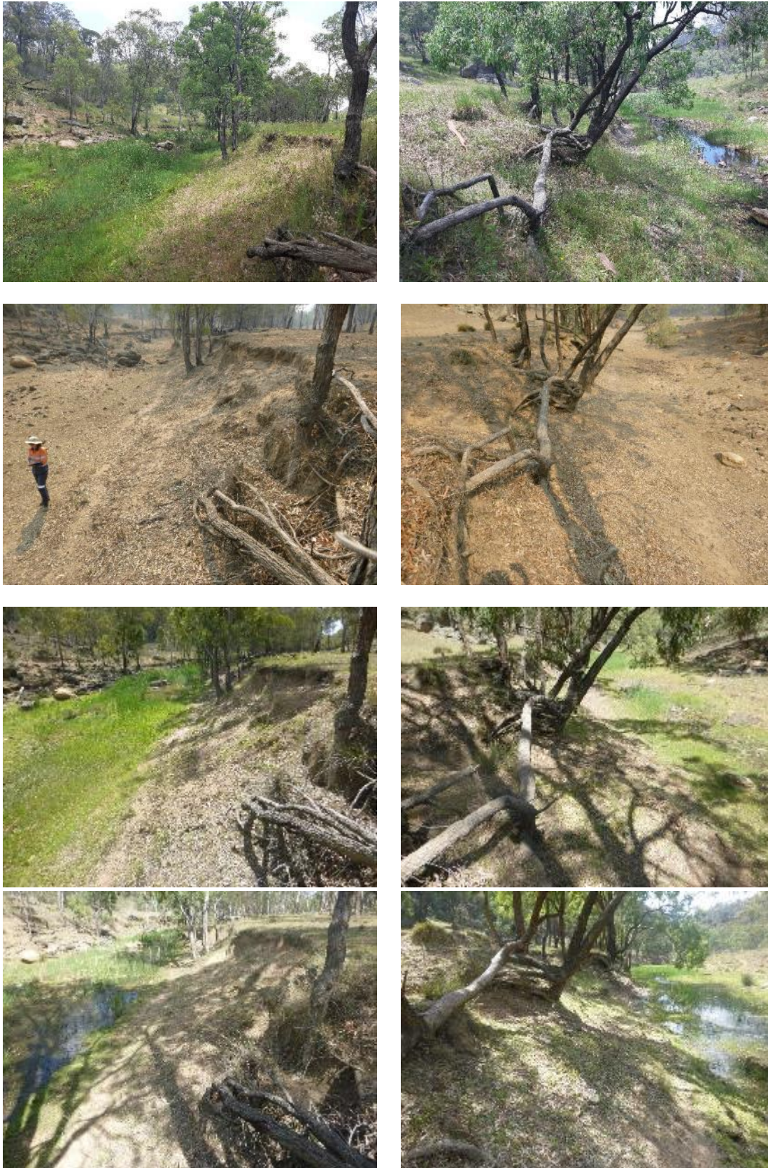
Figure B - 48: Wck48 site photos clockwise from top left: 2020 upstream, 2020 downstream, 2019 downstream, 2018 downstream, 2017 downstream, 2017 upstream, 2018 upstream, 2019 upstream
