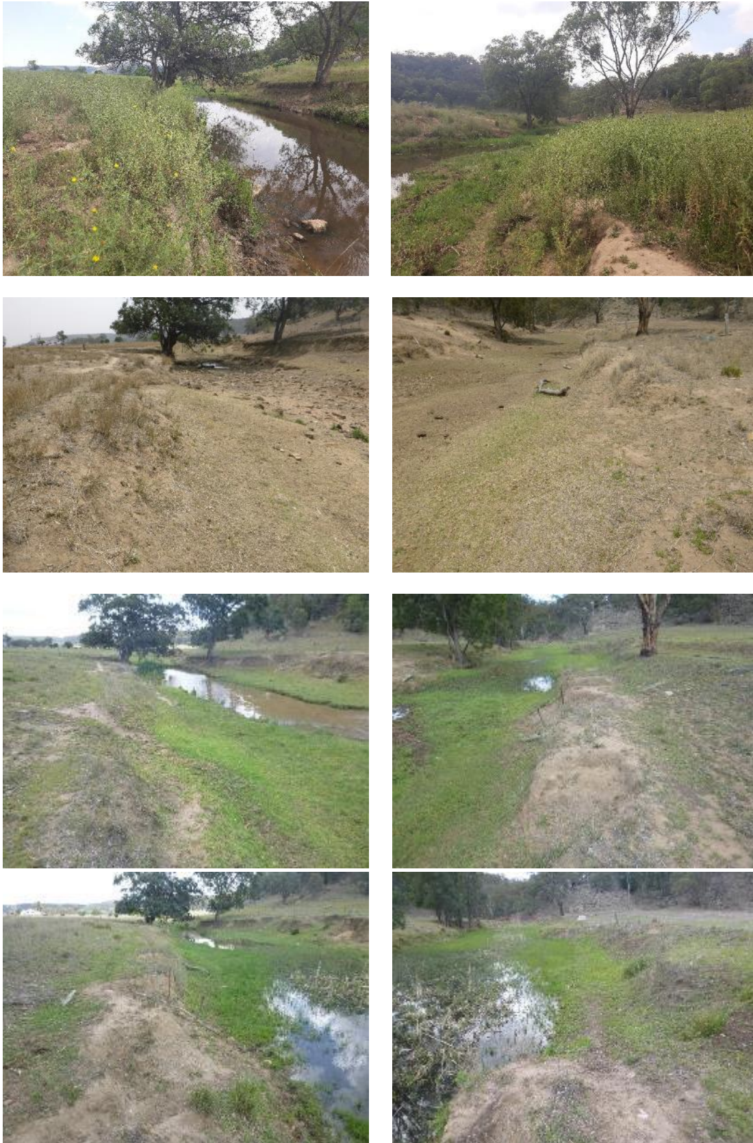
Figure B - 44: Wck44 site photos clockwise from top left: 2020 upstream, 2020 downstream, 2019 downstream, 2018 downstream, 2017 downstream, 2017 upstream, 2018 upstream, 2019 upstream
