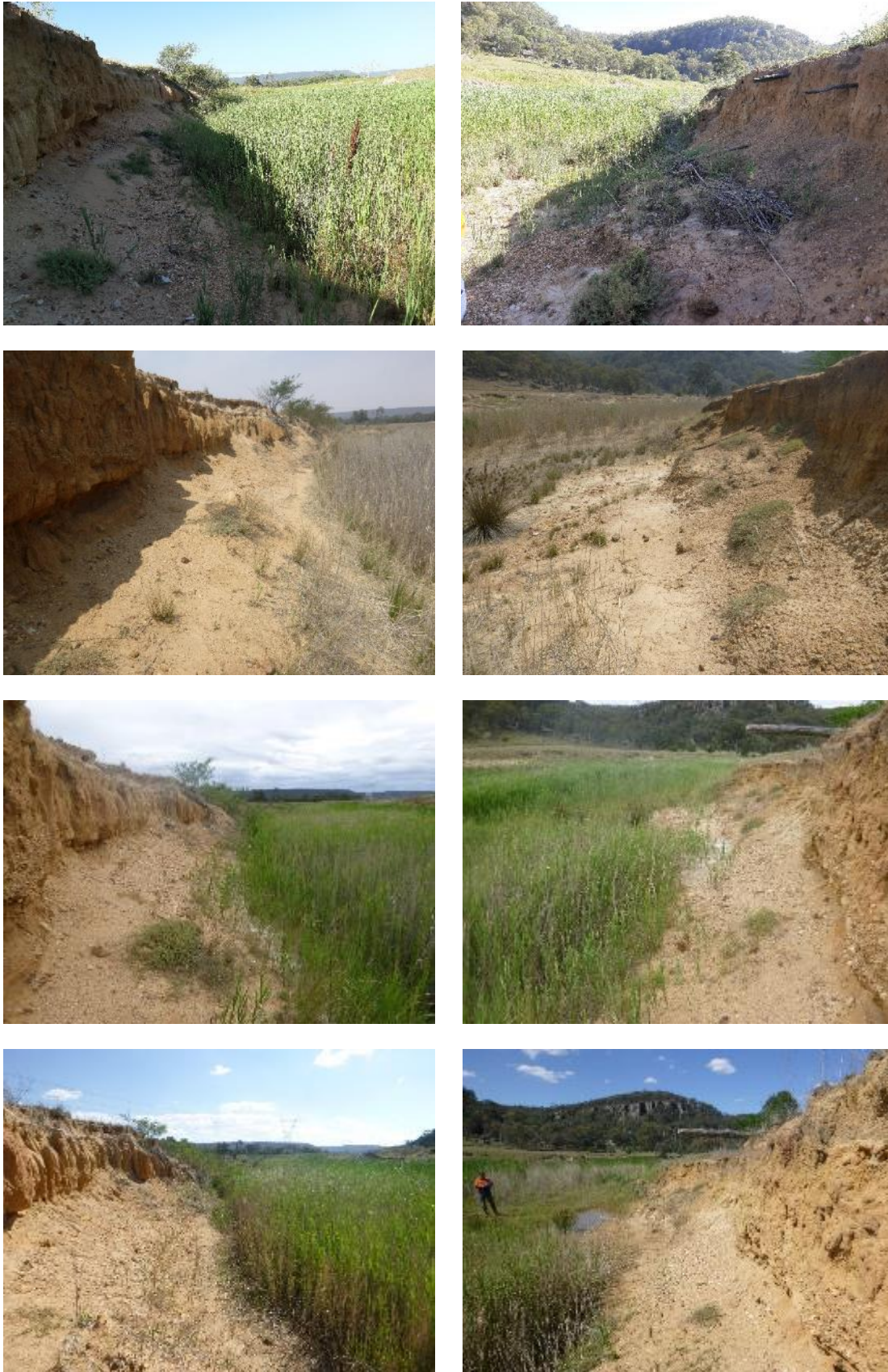
Figure B - 27: Wck27 site photos clockwise from top left: 2020 upstream, 2020 downstream, 2019 downstream, 2018 downstream, 2017 downstream, 2017 upstream, 2018 upstream, 2019 upstream
