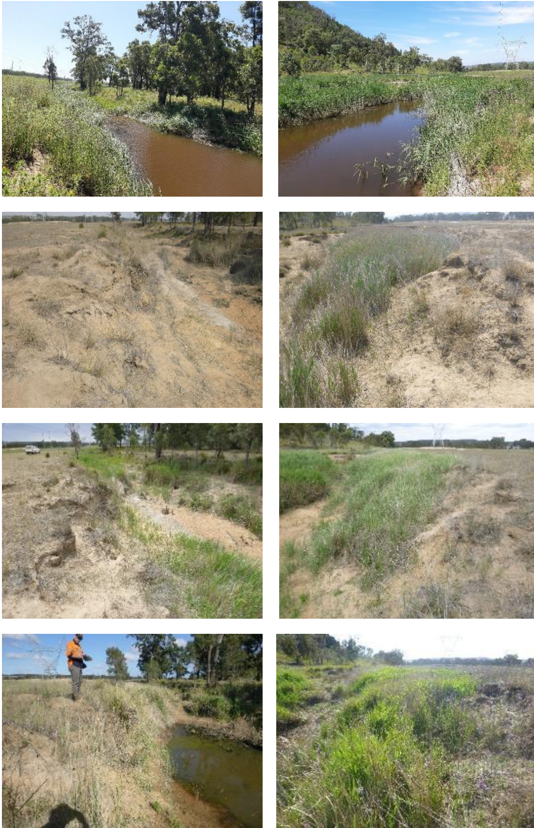
Figure B - 18: WCK18 site photos clockwise from top left: 2020 upstream, 2020 downstream, 2019 downstream, 2018 downstream, 2017 downstream, 2017 upstream, 2018 upstream, 2019 upstream
