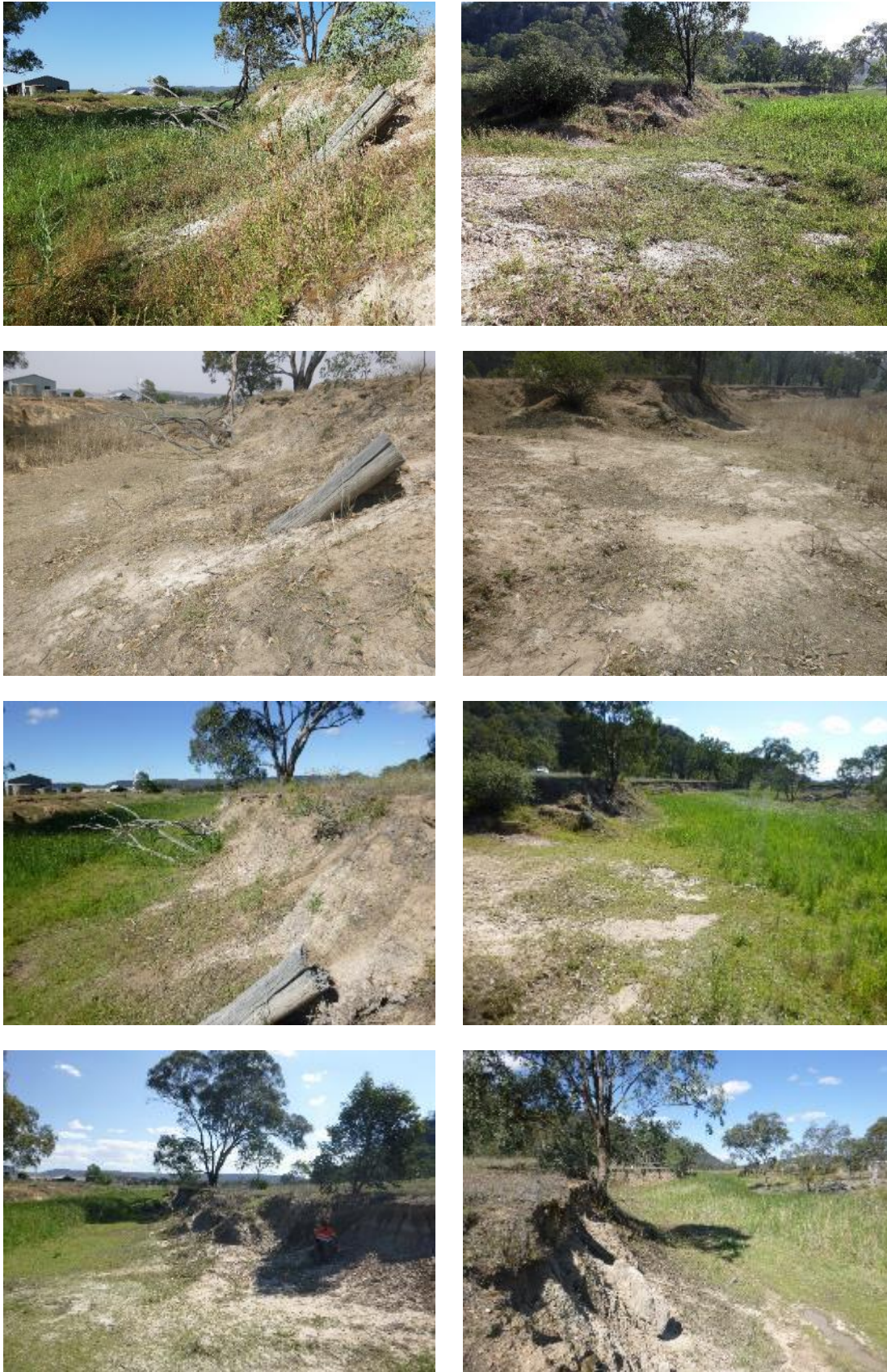
Figure B - 28: Wck28 site photos clockwise from top left: 2020 upstream, 2020 downstream, 2019 downstream, 2018 downstream, 2017 downstream, 2017 upstream, 2018 upstream, 2019 upstream
