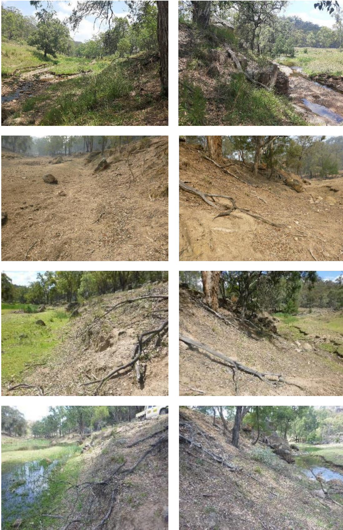
Figure B - 49: Wck49 site photos clockwise from top left: 2020 upstream, 2020 downstream, 2019 downstream, 2018 downstream, 2017 downstream, 2017 upstream, 2018 upstream, 2019 upstream
