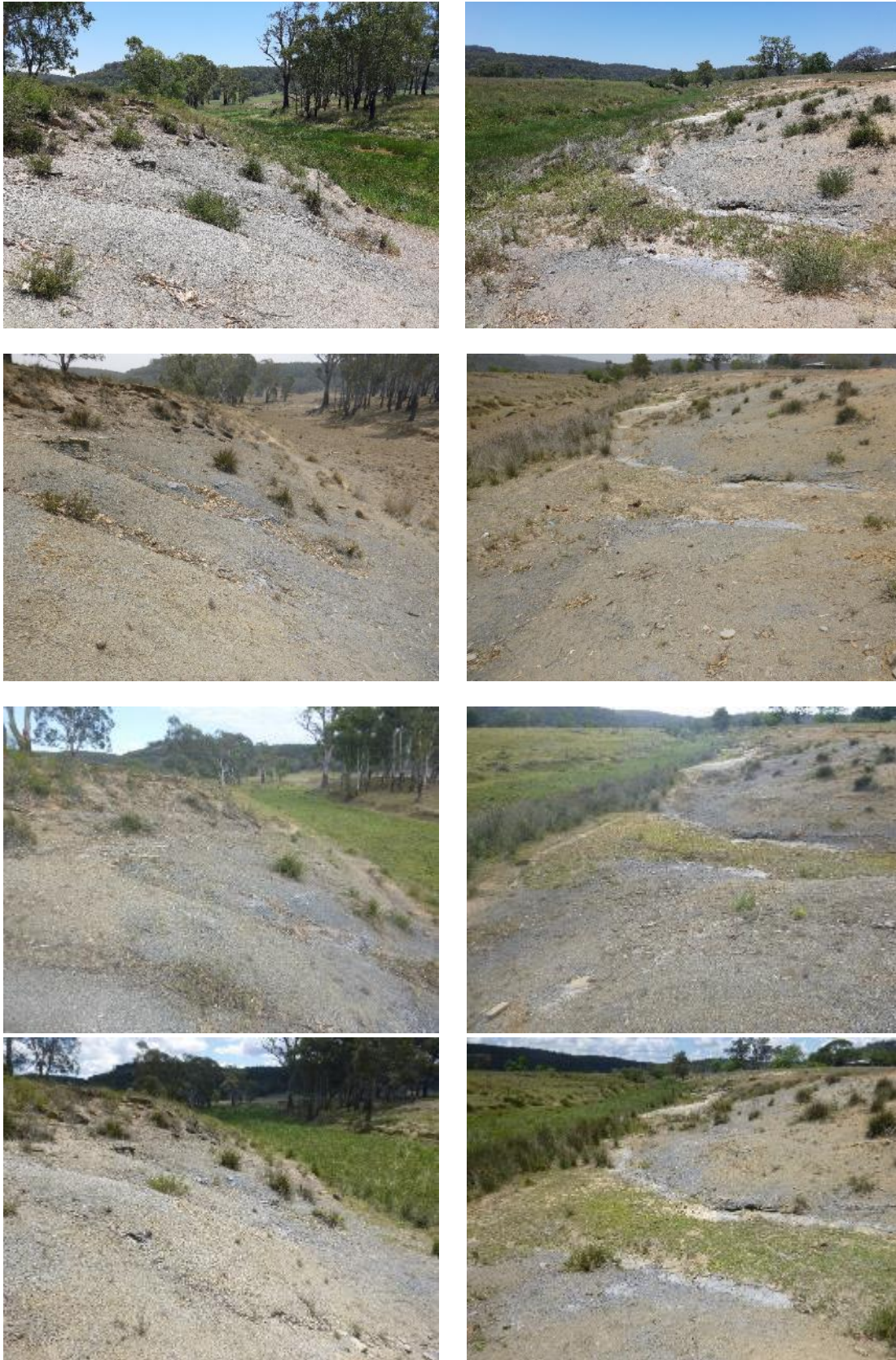
Figure B - 40: Wck40 site photos clockwise from top left: 2020 upstream, 2020 downstream, 2019 downstream, 2018 downstream, 2017 downstream, 2017 upstream, 2018 upstream, 2019 upstream
