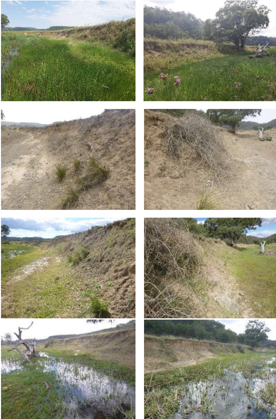
Figure B - 43: Wck43 site photos clockwise from top left: 2020 upstream, 2020 downstream, 2019 downstream, 2018 downstream, 2017 downstream, 2017 upstream, 2018 upstream, 2019 upstream
