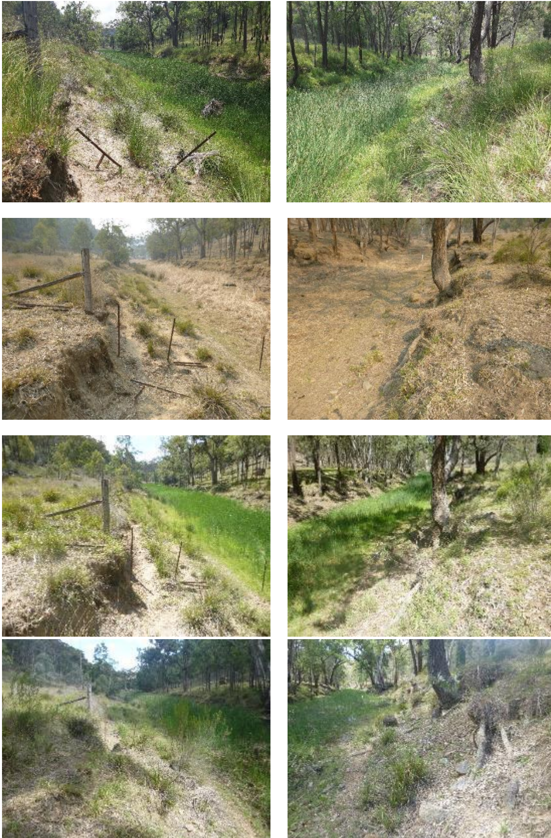
Figure B - 47: Wck47 site photos clockwise from top left: 2020 upstream, 2020 downstream, 2019 downstream, 2018 downstream, 2017 downstream, 2017 upstream, 2018 upstream, 2019 upstream
