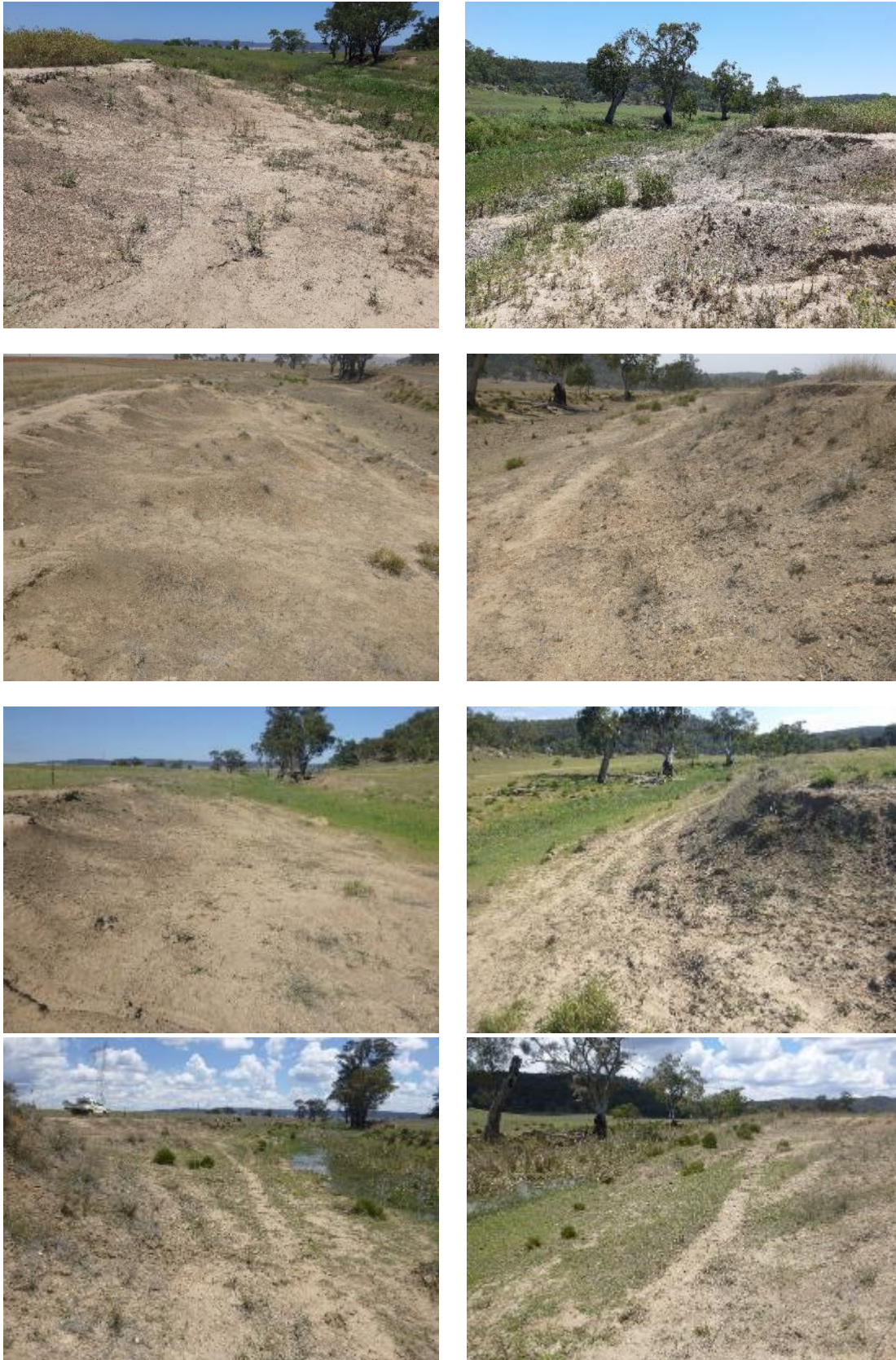
Figure B - 37: Wck37 site photos clockwise from top left: 2020 upstream, 2020 downstream, 2019 downstream, 2018 downstream, 2017 downstream, 2017 upstream, 2018 upstream, 2019 upstream
