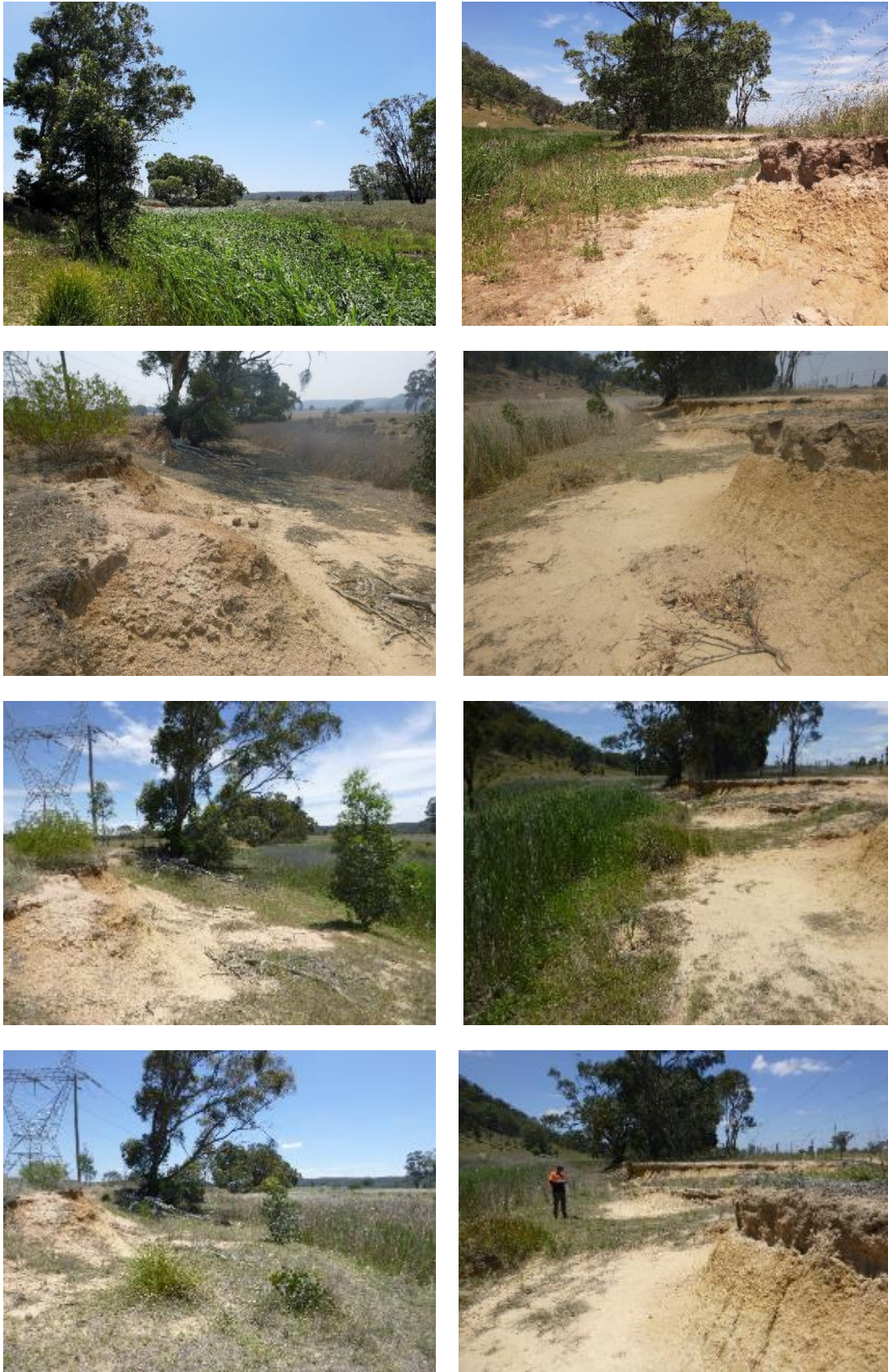
Figure B - 9: Wck9 site photos clockwise from top left: 2020 upstream, 2020 downstream, 2019 downstream, 2018 downstream, 2017 downstream, 2017 upstream, 2018 upstream, 2019 upstream
