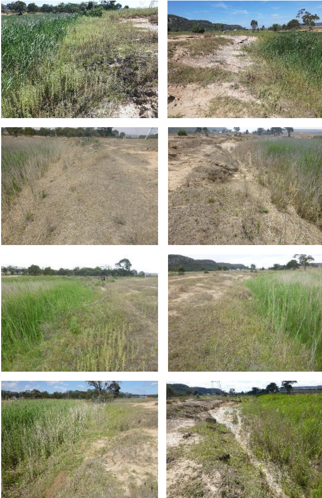
Figure B - 25: Wck25 site photos clockwise from top left: 2020 upstream, 2020 downstream, 2019 downstream, 2018 downstream, 2017 downstream, 2017 upstream, 2018 upstream, 2019 upstream
