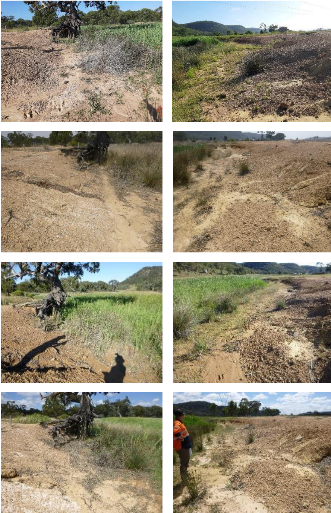
Figure B - 24: Wck24 site photos clockwise from top left: 2020 upstream, 2020 downstream, 2019 downstream, 2018 downstream, 2017 downstream, 2017 upstream, 2018 upstream, 2019 upstream
