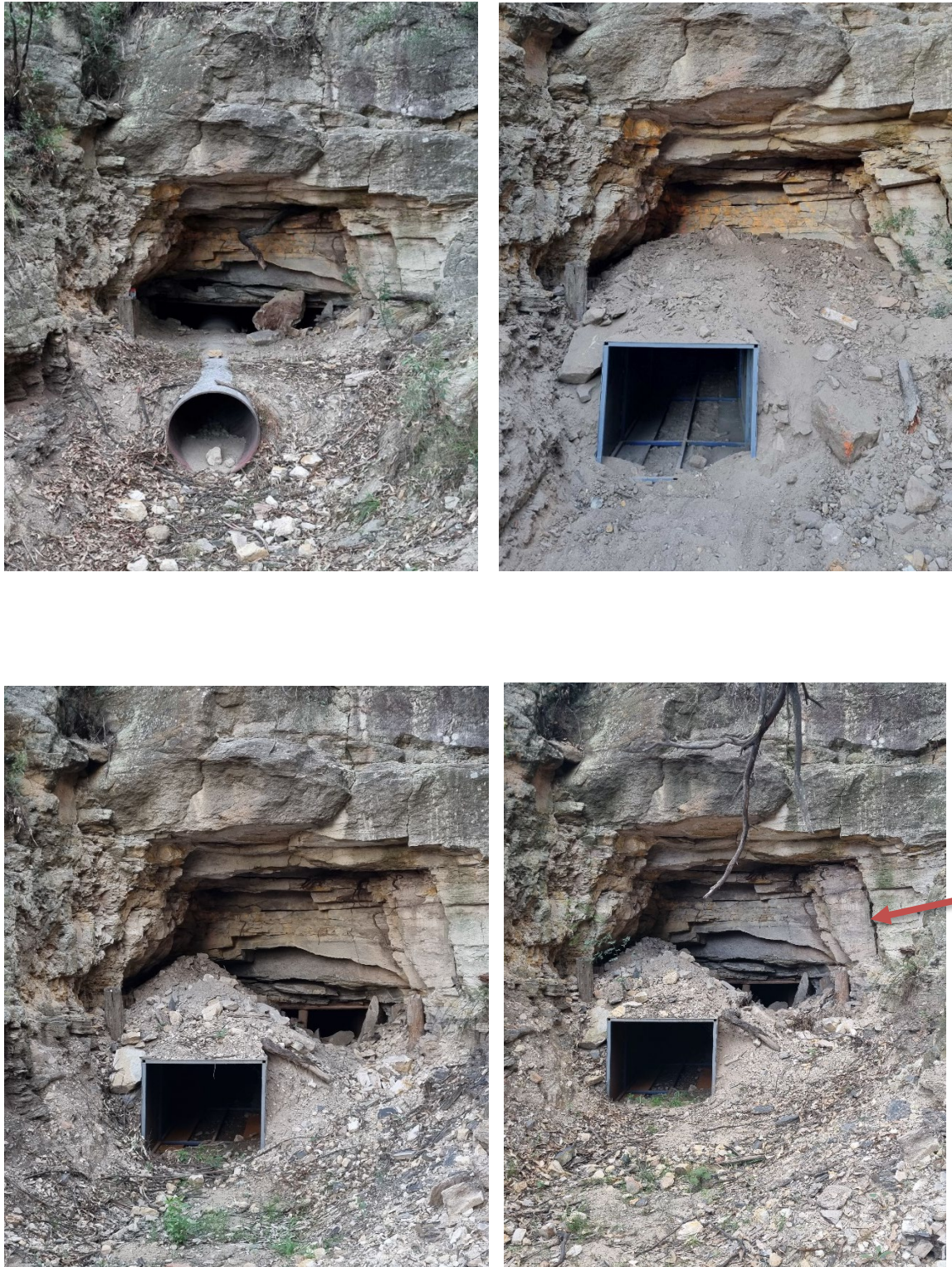
Plate 5-2: Monitoring photos of adit entrance pre culvert installation (March 2023 – top left), afternoon of installation (April 2023 – top right), nine months after installation (January 2024 – bottom left), and 20 months after installation (December 2024 – bottom right). This shows progression of pipe to tunnel with
