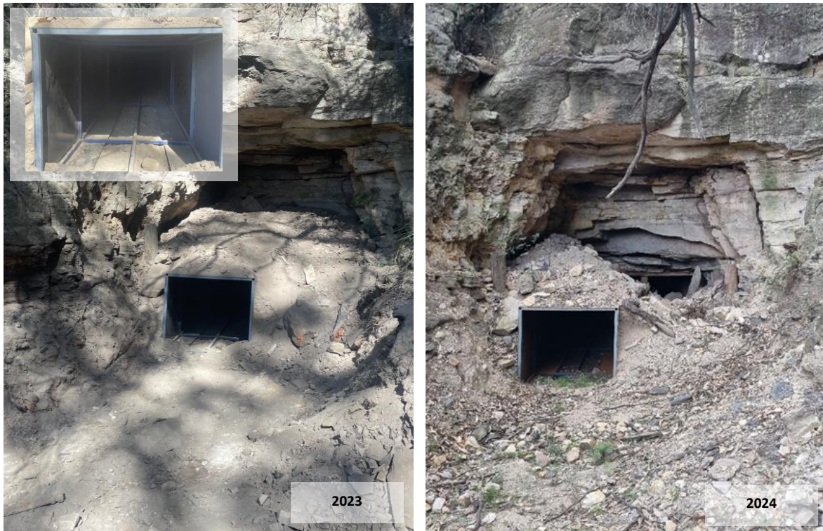
Photo 3 Upgrades to the Bat Adit Culvert in 2023 and Adit Condition in 2024
