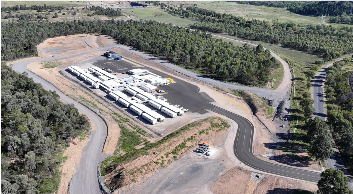
Photo 1 On Site Accommodation Facility
