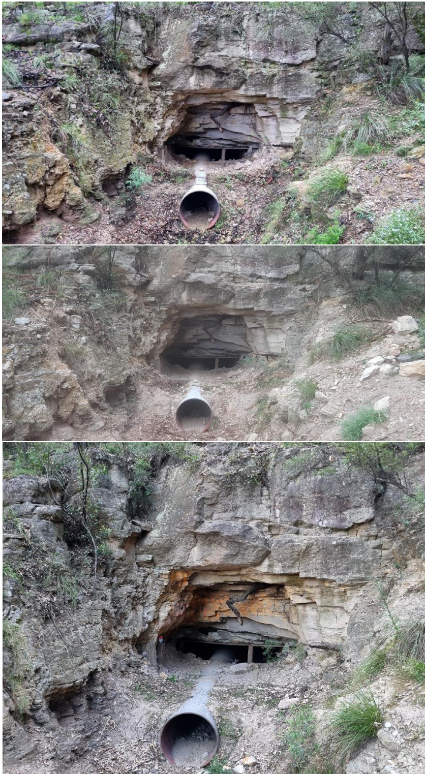
Plate 5-A: Periodic monitoring photo of adit entrance from February 2021 (top), January 2022 (middle) and December 2022 (bottom) showing lack of substantial change
