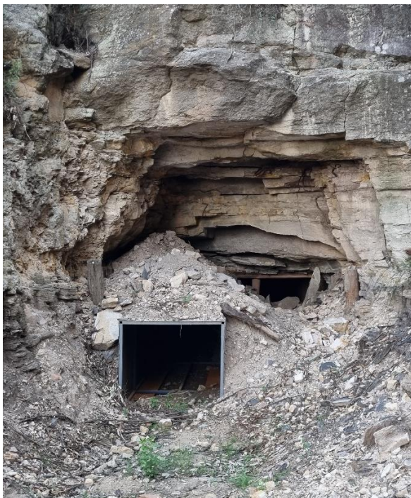
Plate 5-B: Monitoring photos of adit entrance pre culvert installation (March 2023 – top left), afternoon of installation (April 2023 – top right), nine months after installation (January 2024 – bottom left), and 20 months after installation (December 2024 – bottom right). This shows progression of pipe to tunnel with small aperture, tunnel with large aperture. Large crack forming on western side shown with red arrow.
