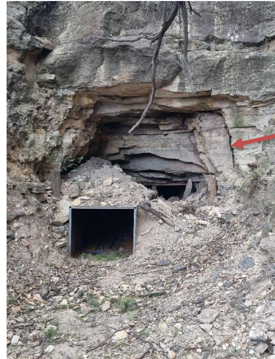
Plate 5-B: Monitoring photos of adit entrance pre culvert installation (March 2023 – top left), afternoon of installation (April 2023 – top right), nine months after installation (January 2024 – bottom left), and 20 months after installation (December 2024 – bottom right). This shows progression of pipe to tunnel with small aperture, tunnel with large aperture. Large crack forming on western side shown with red arrow.
