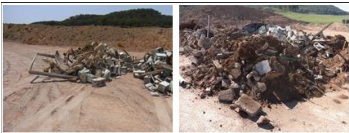
Plate 1 Mogo Road properties demolition material (awaiting in-pit disposal)
