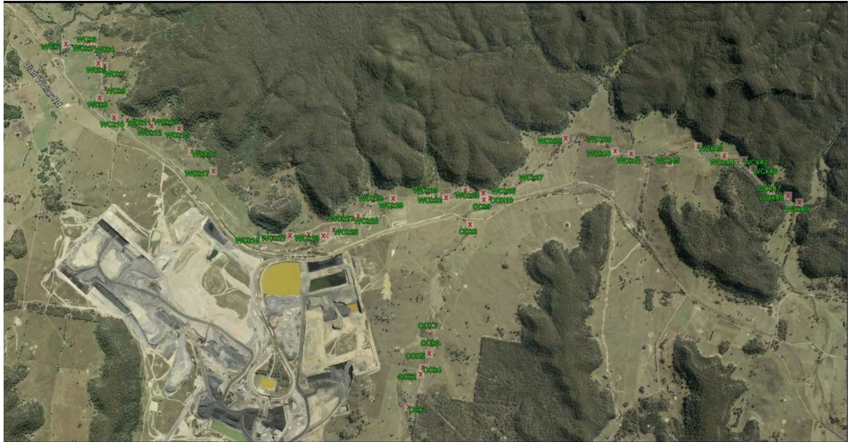
FIGURE 1 - WILPINJONG CREEK AND CUMBO CREEK SURVEY LOCATIONS
