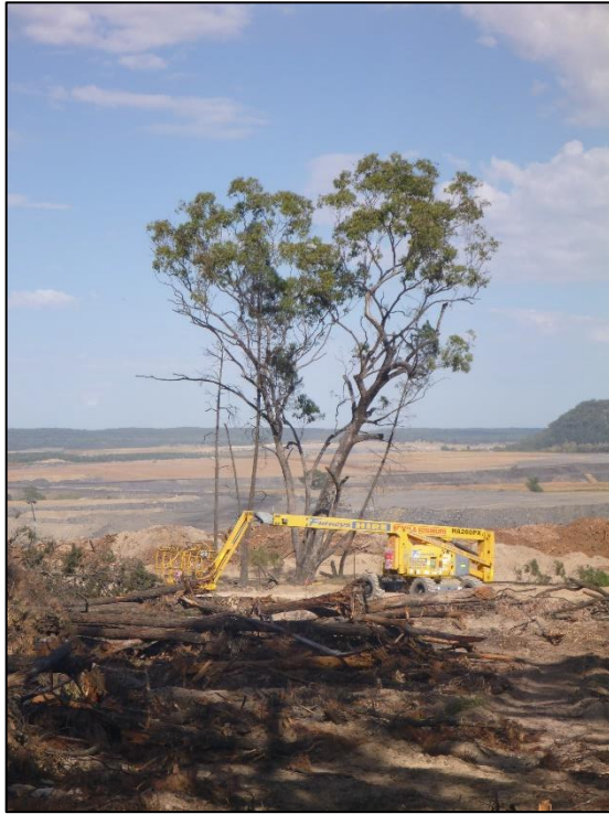
WCP 99 prior to limb removal looking west
