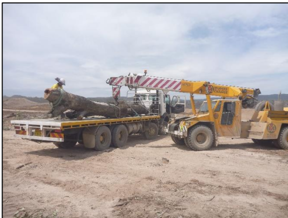
WCP 95 removal onto truck
