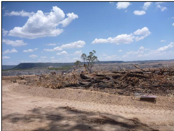
WCP 95 during limb removal looking west
