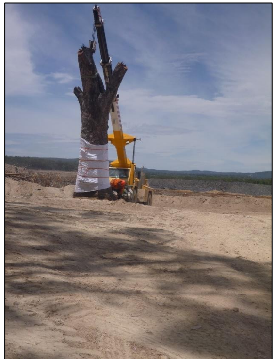
WCP94 wrapped in geotextile being removed using franna
