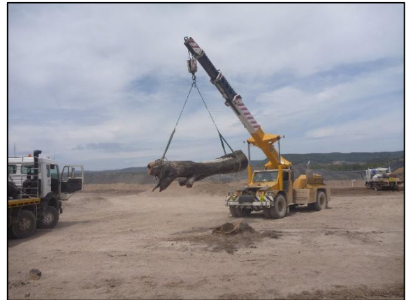
WCP 95 removal by franna
