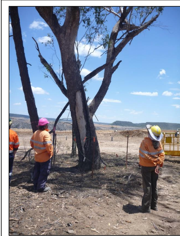
WCP 95 prior to limb removal looking west
