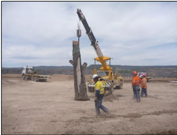
WCP 95 removal by franna
