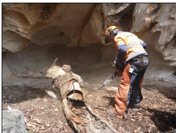
Cutting and removal of remnant stump, looking E.
