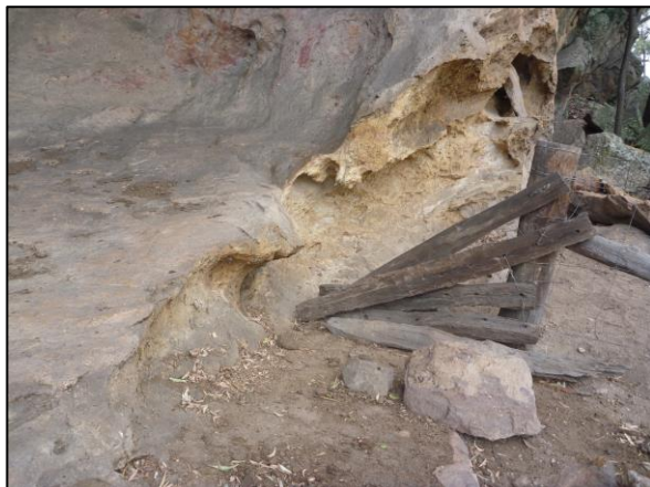
View of end post and rails at shelter end of fenceline, looking N.
