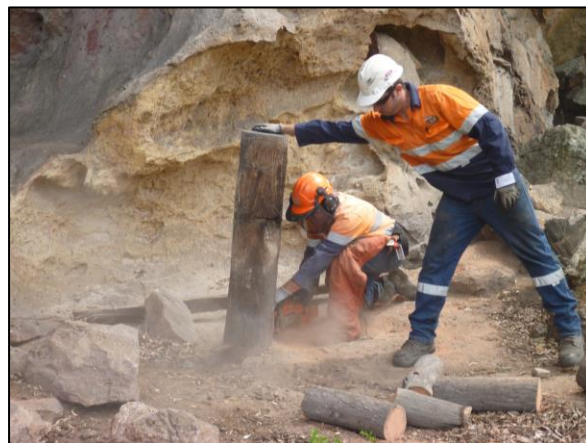
Cutting of end post at base, (portion below ground left in situ ).
