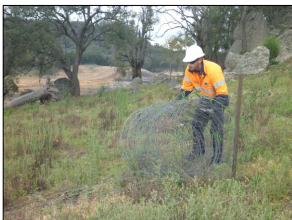
Removal of wire mesh.
