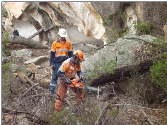
Cutting and removal of tree fall near and downslope of S end of shelter, looking NE.
