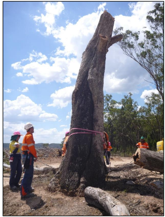
WCP94 after limb removal - north
