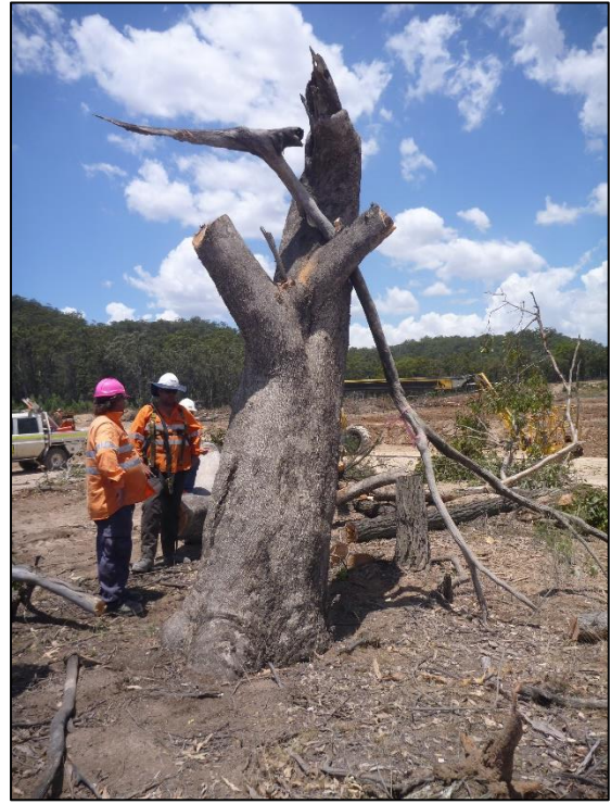
WCP 95 following limb removal looking east
