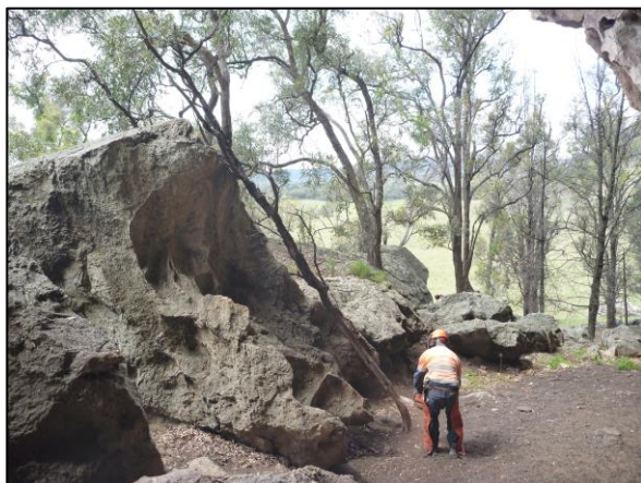
Felling and removal of dead tree situated within the shelter space and behind the dripline, looking SE. Note dead standing trees at far right.
