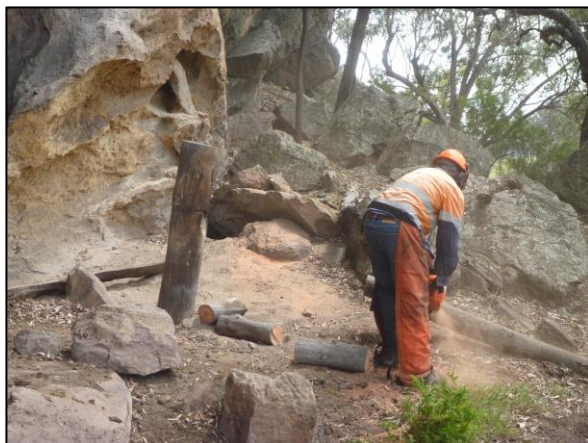
Removal of strainer post and rails.
