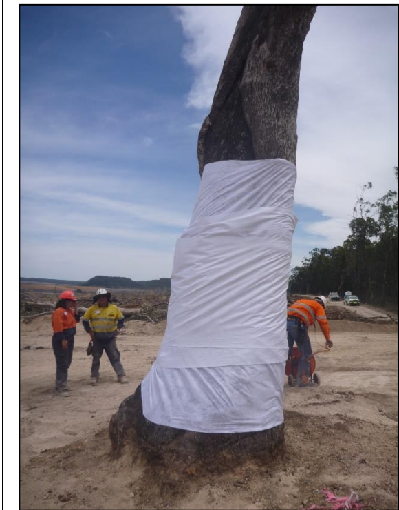
WCP94 wrapped in geotextile
