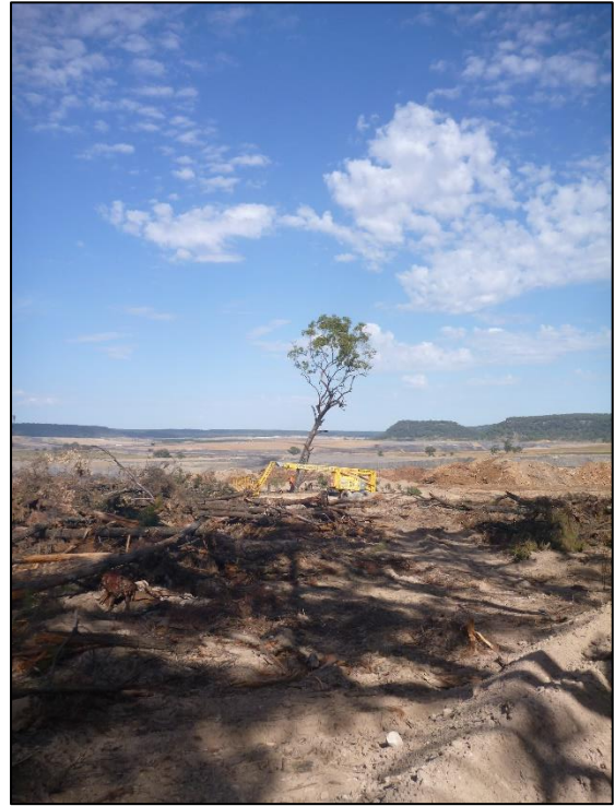
WCP 99 during limb removal looking west
