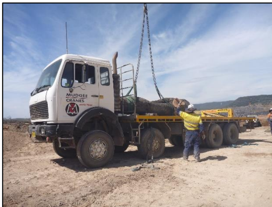
WCP 99 removal onto truck
