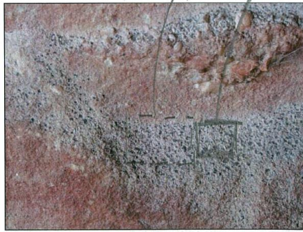
Figure 4.10 General view of lichen growing on dust deposits on an upward facing micro-ledge (photo 404)
