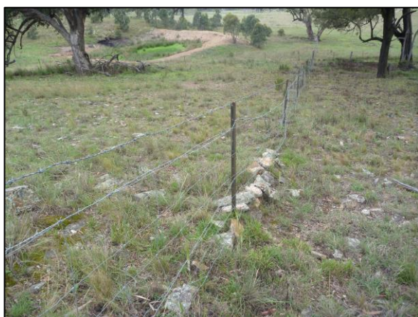
View of downslope end of fenceline prior to demolition, looking E.
