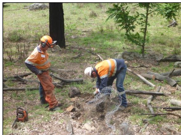
Removal of collapsed wire mesh along older former fenceline.
