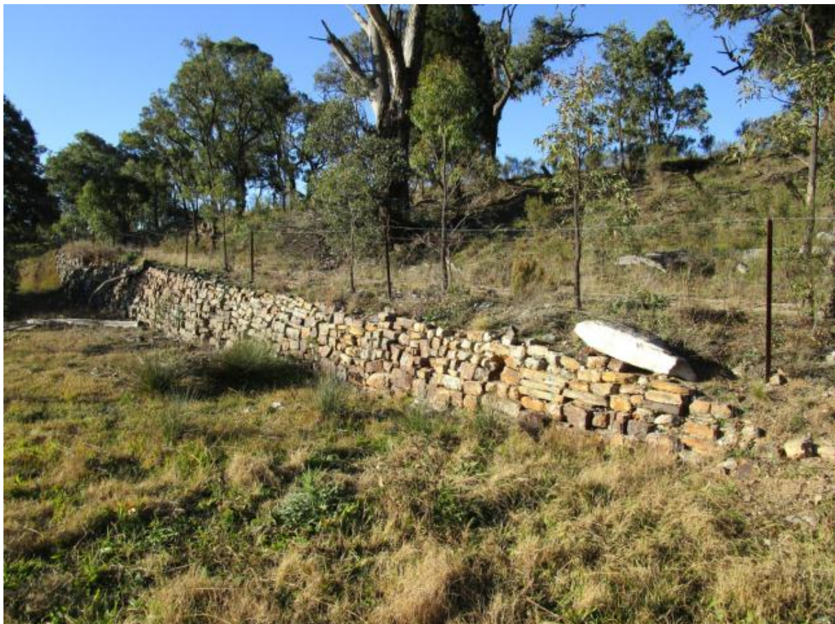
Plate 2 Road Embankment (Niche, 2015)
