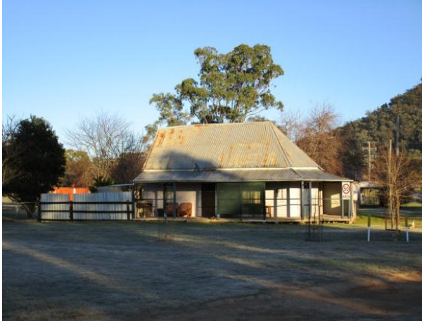
Plate A2-7 Former Mason's Store (Niche, 2015)
