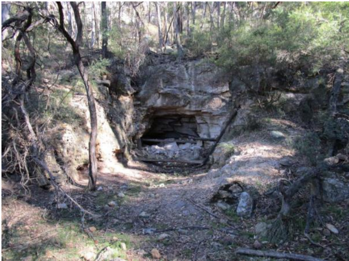
Plate 1 Historical Shale Oil Mine Adit (Niche, 2015)
