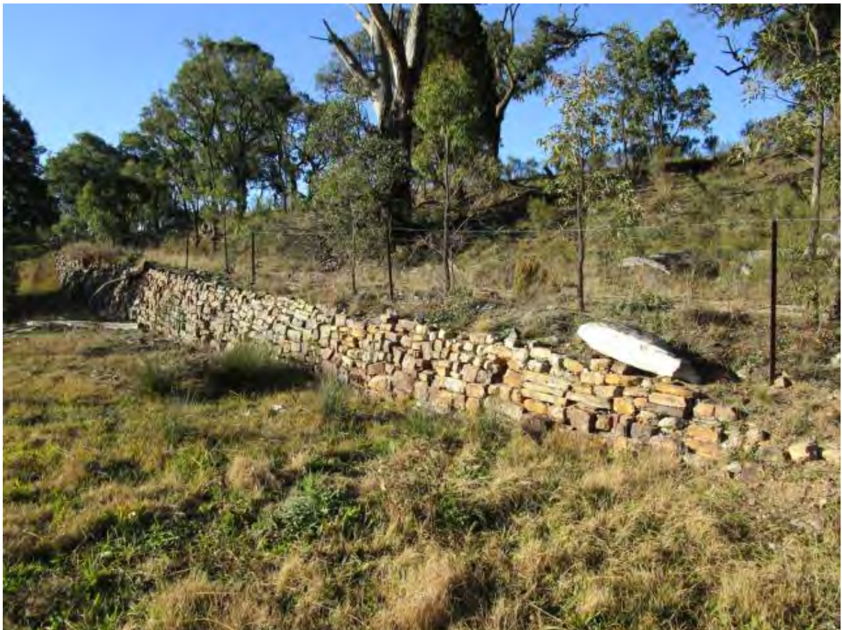
Plate 2 Road Embankment (Niche, 2015)
