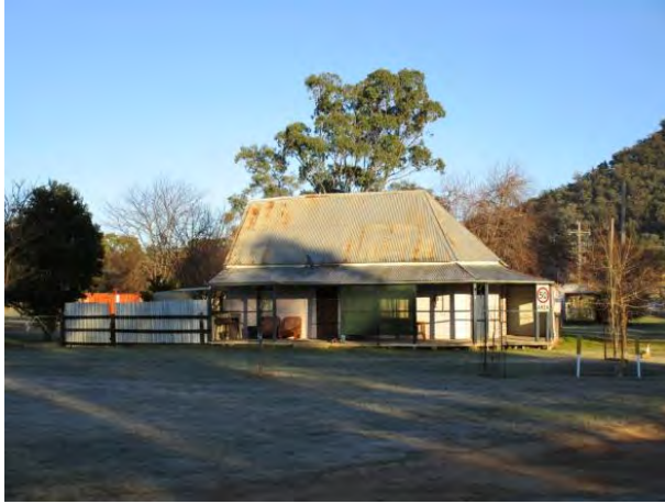
Plate A2-7 Former Mason's Store (Niche, 2015)
